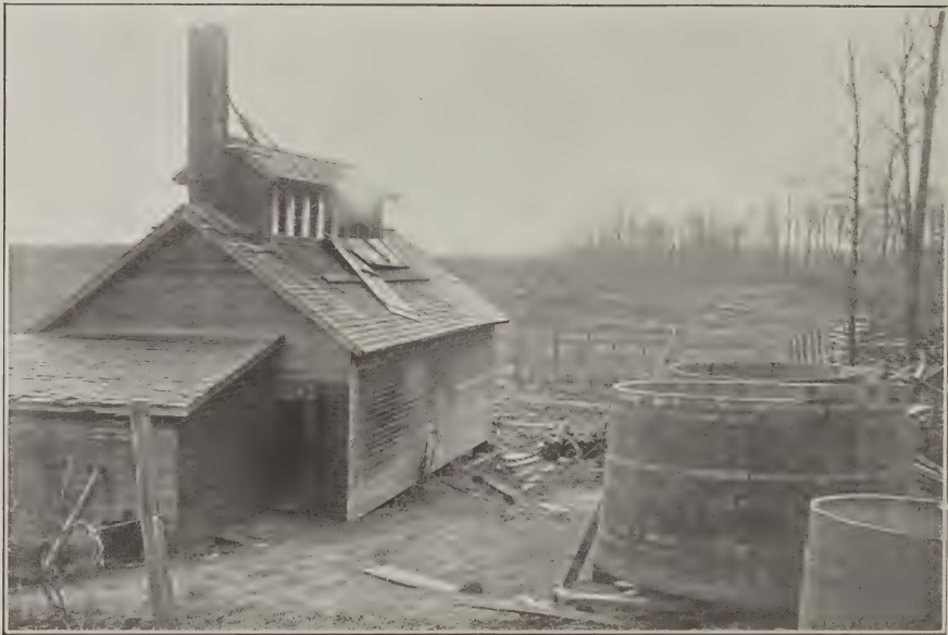
21. Maple sugar industry. A modern sugar house with storage tanks. Underground connection with evaporating pan. Covers of storage tanks not shown.
