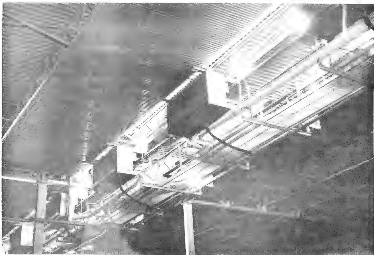
FIGURE 6.—Looking up at unit coolers, pipes, and catwalk located overhead in the center of a cold-storage room.
