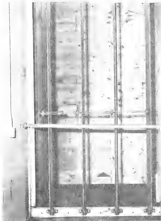
FIGURE 11.—Open reversing dampers in a large air duct.
