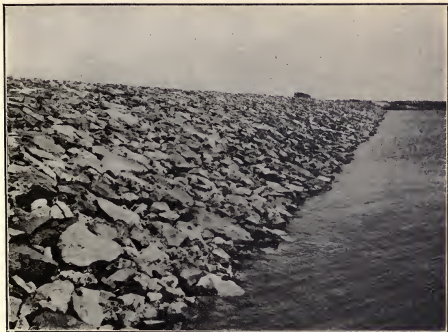
FIG. 33.—Riprapped slope, Minidoka Dam, Snake River, Idaho.
