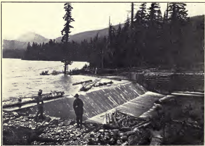
FIG. 2.—THE COMPLETED DAM, LAKE KEECHELUS, WASH., SHOWING SPILLWAY AND BULKHEAD.
