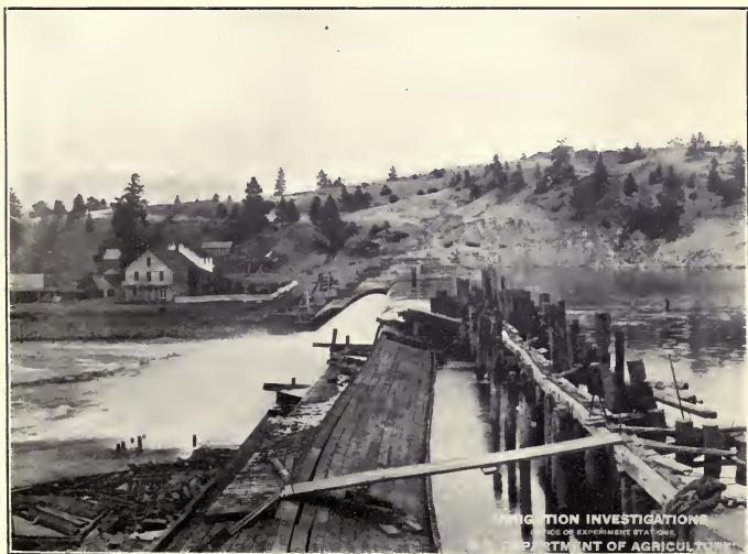
FIG. 2.—CANYON FERRY DAM, BEFORE RECONSTRUCTION.
