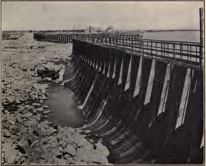
FIG. 36.—Spillway, Minidoka Dam, Idaho (U. S. Reclamation Service).
