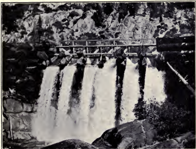
FIG. 1.—WASTEWAY, MIDDLE DAM, SOUTH FORK STANISLAUS RIVER, CAL.
