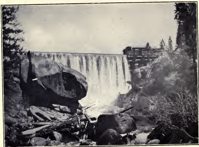
FIG. 1.—LYONS DAM, SOUTH FORK STANISLAUS RIVER, CAL.
