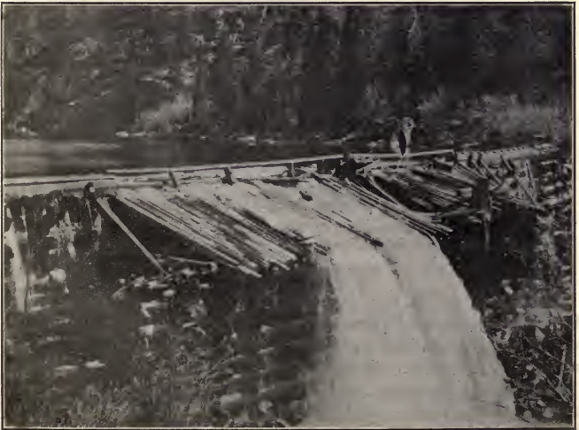
FIG. 8.—Lower Strawberry Dam, South Fork Stanislaus River, Cal.
