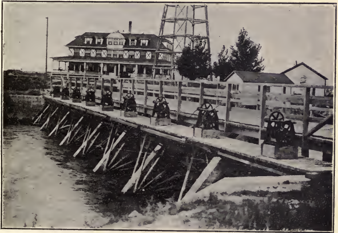
FIG. 31.—Headgates, Twin Falls Canal system, South Side, at Milner, Idaho.
