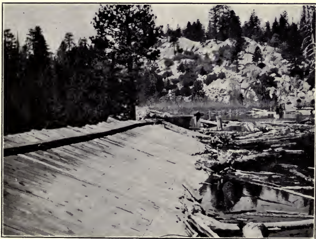
FIG. 2.—PLANKING ON UPSTREAM FACE OF MIDDLE DAM, SOUTH FORK STANISLAUS RIVER, CAL.
