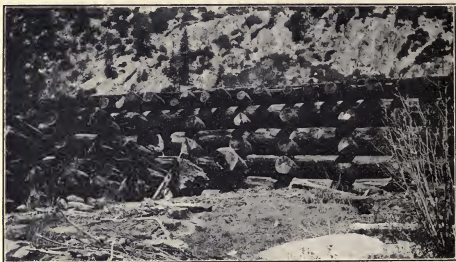
FIG. 5.—Middle Dam, South Fork Stanislaus River, Cal., showing manner of laying logs from the reservoir site. The site was not thoroughly cleared, however, only the best timber suitable for the construction of the dam being used. This standing timber is rotting at the water's edge and
