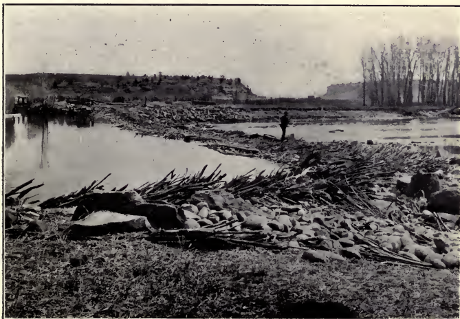
FIG. 2.—A BRUSH DAM ON THE YELLOWSTONE RIVER.
