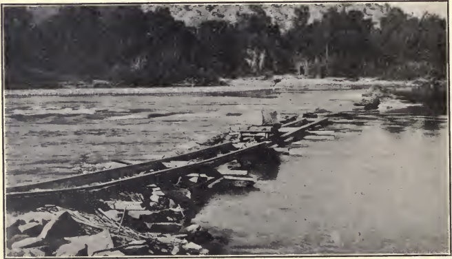
FIG. 1.—Repairing a brush dam on the Yellowstone River.
