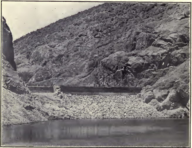
FIG. 2.—SAME, SHOWING STEEL CORE PROJECTING, AND SPILLWAY ON LEFT, AUGUST, 1900.
