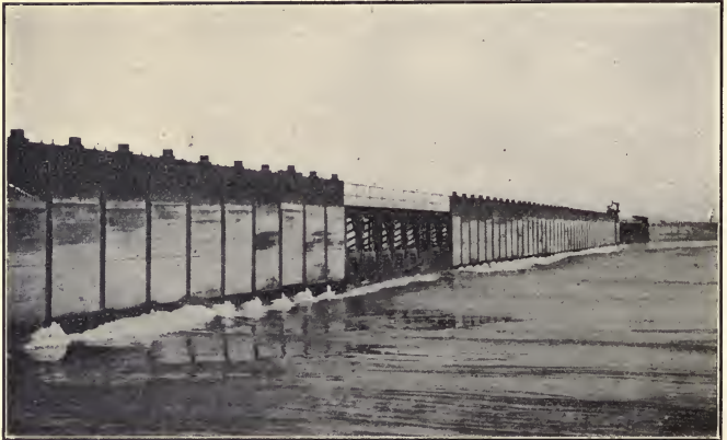
FIG. 29.—Gates in Milner Dam, Snake River, Idaho. At times of high water these gates are raised to regulate flow in canals.
