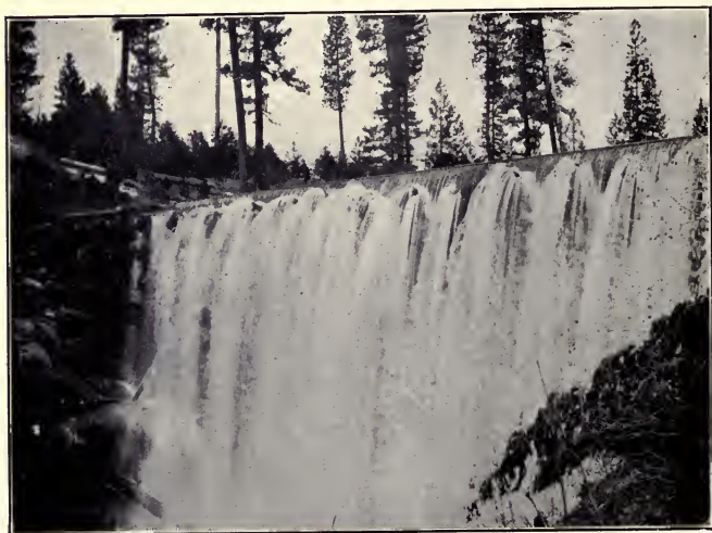
FIG. 2.—LYONS DAM, ANOTHER VIEW.
