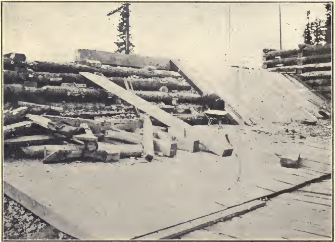
FIG. 12.—Lake Keechelus Dam, apron and spillway under construction, crest log in place and apron completed on east end.
