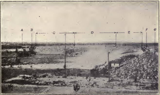
FIG. 28.—General view of Milner Dam, Snake River, Idaho: A, Control or wastegates on canal; B, Headgates, North Side Canal; C, North dam, length 340 feet on top; D, Spillway, concrete apron; E, Middle dam, length 335 feet on top; F, Regulating gates (99); G, South dam, length 560 feet on top. Total length of structure 2,100 feet.
