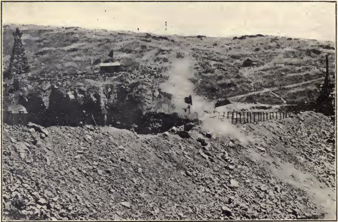
FIG. 25.—Lower Otay Dam—two cableways delivering rock from quarry.
