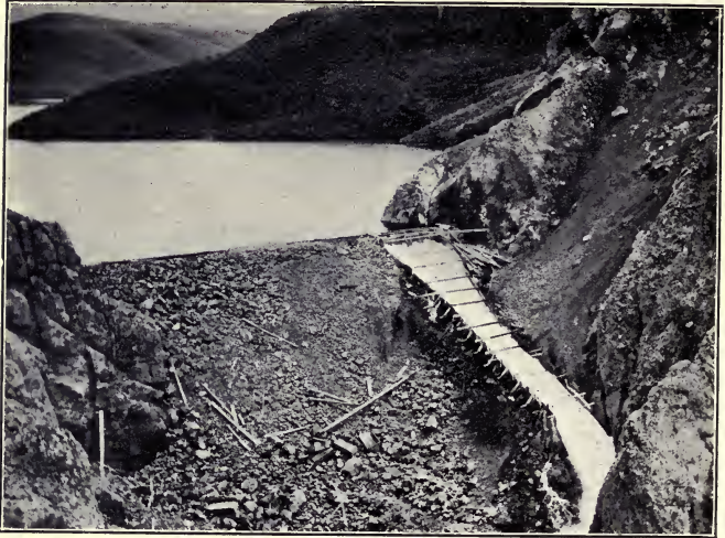
FIG. 1.—EAST CANYON DAM, UTAH, SHOWING TEMPORARY SPILLWAY.
