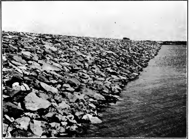
FIG. 33.—Riapped slope, Minidoka Dam, Snake River, Idaho.
