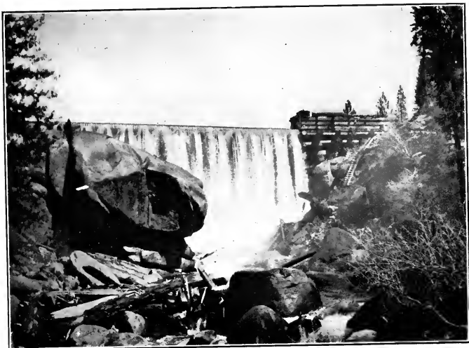
FIG. 1.—LYONS DAM, SOUTH FORK STANISLAUS RIVER, CAL.
