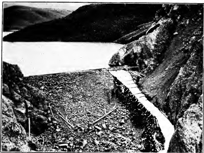
FIG. 1.—EAST CANYON DAM, UTAH, SHOWING TEMPORARY SPILLWAY.
