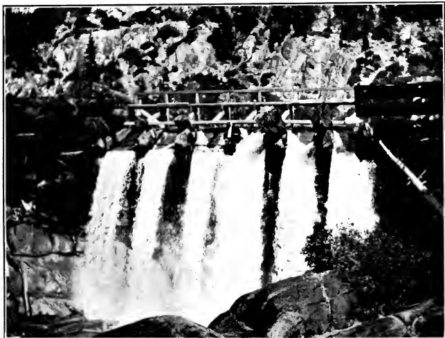
FIG. 1.—WASTEWAY, MIDDLE DAM, SOUTH FORK STANISLAUS RIVER, CAL.
