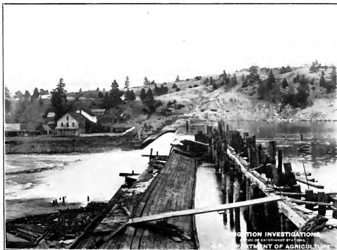
FIG. 2.—CANYON FERRY DAM, BEFORE RECONSTRUCTION.
