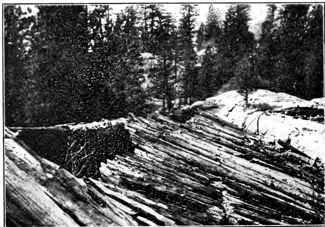
FIG. 6.—Abandoned portion of Middle Dam, illustrating the placing of logs on upstream slope of continuous-crib dams.
