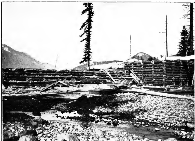
FIG. 1.—LAKE KEECHELUS CRIB DAM DURING CONSTRUCTION, DOWNSTREAM VIEW.
