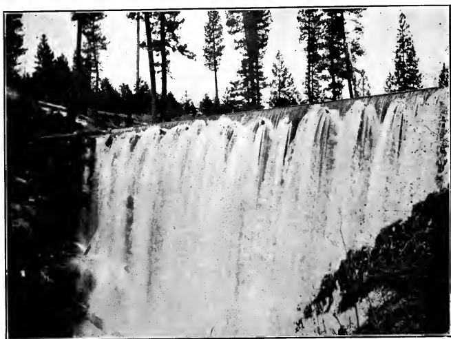
FIG. 2.—LYONS DAM, ANOTHER VIEW.
