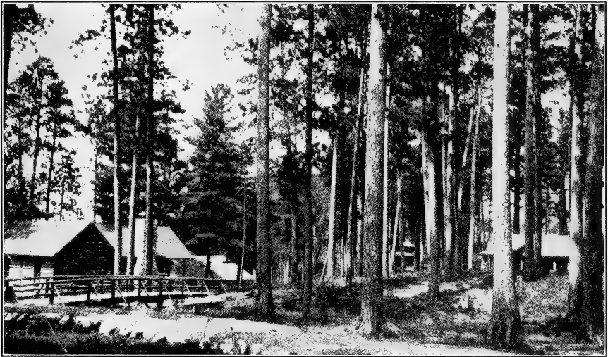
FIG. 91. Cottages at Douglas Lodge, Itasca State Park.
