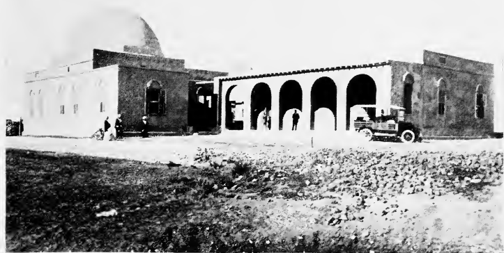
Chicago House, Luxor, Egypt
