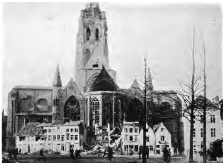
Cathedral Saint-Walburga, showing damage done by shell fire. This church was first built in the thirteenth century and later added to in the sixteenth century. Audenarde, Belgium.
