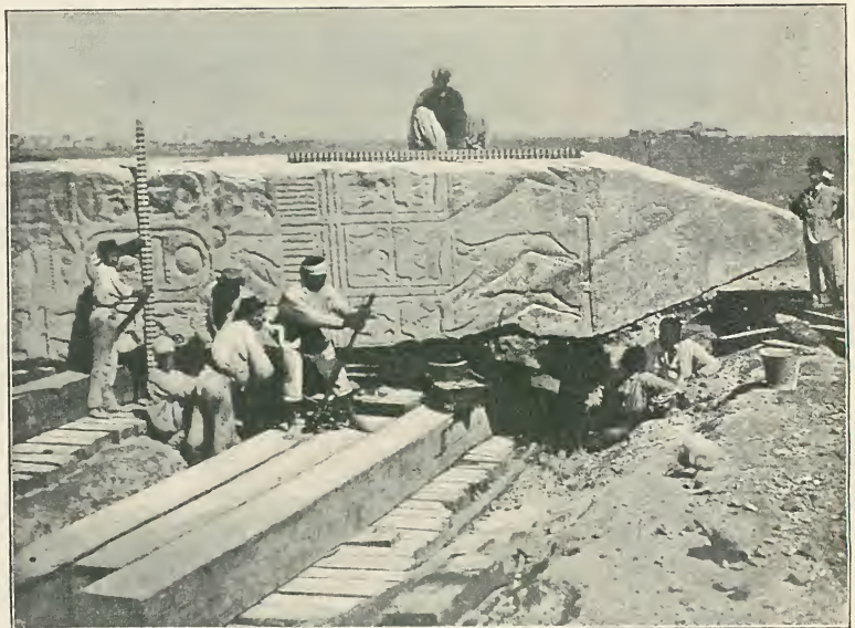
From a] PRISING UP THE NEEDLE, IN ORDER TO BUILD THE FRAMEWORK UNDER IT. [Photo.
