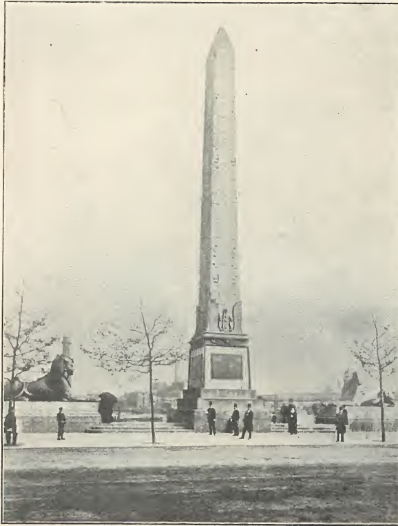
ON THE THAMES EMBANKMENT.
