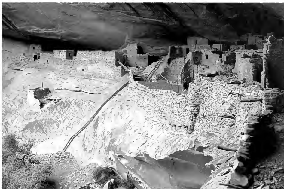
Figure 5-21. Access into Kiet Siel. The Park Service ladder visible in the left center of the photograph is approximately parallel to the prehistoric hand- and toeholds leading into the site.
