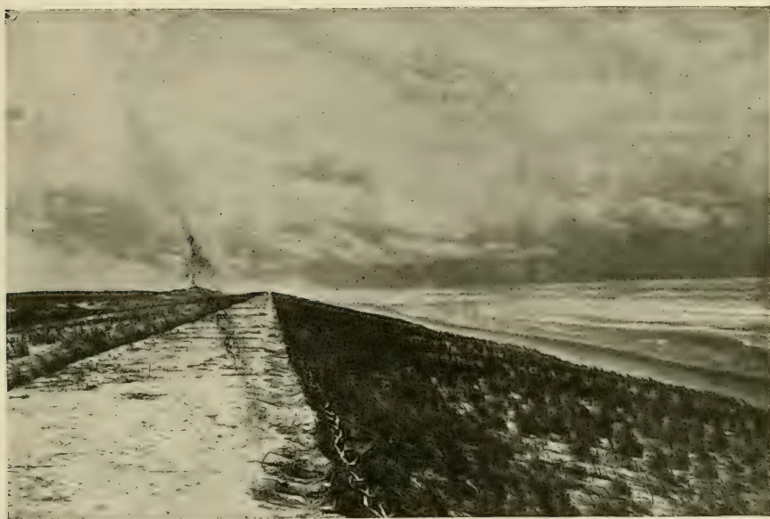
FIG. 15. — Protection dune at Lacanau-Océan in State forest of Lacanau (Gironde). The sand is held in place by planting maram grass on the wind-swept dunes.
