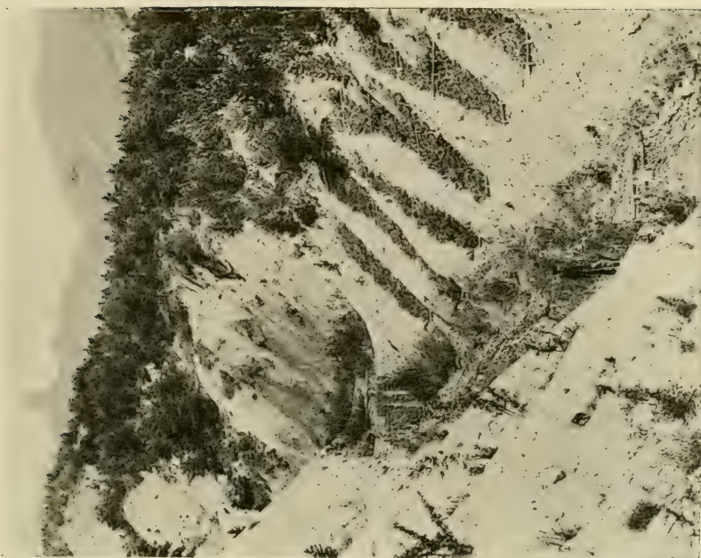
FIG. 10 (d). — Wattle work on small side gullies and masonry dam in main ravine in Ubaye area (Basses-Alpes). (French official photograph.)
