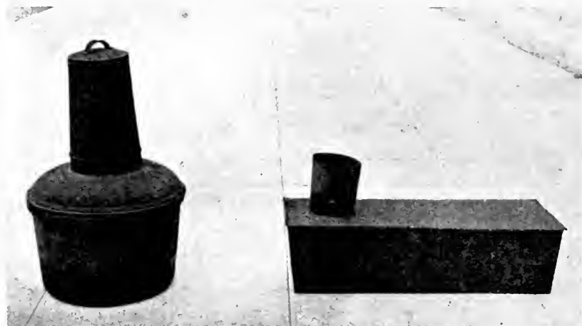
Fig. 8.—On right one of the types of orchard oil heaters very commonly used at the time of the 1913 freeze, having a sliding top and with openings on the side for air draft. On left one of the best orchard heaters that has been perfected since 1913. The smoke stack and drafts are hidden by the cover which is lifted off when heater is lighted. Photo by Barrett.
