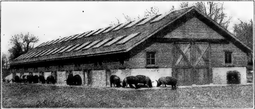
Figure 206.—An Iowa piggyery, showing concrete foundation and outside feeding platform. Note the large amount of sunlight provided through the roof. Photograph by E. J. Hall.
