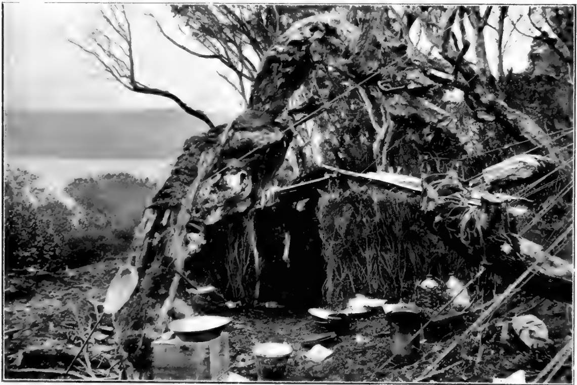
FIG. 11. -HUT BUILT BY SHIPWRECKED SAILORS OF THE "ANJOU" IN CARNLEY HARBOUR. Used as camp kitchen by the Auckland Island party.
