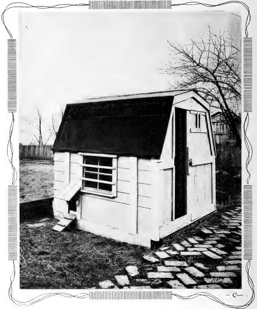
PIANO BOX POULTRY HOUSE
