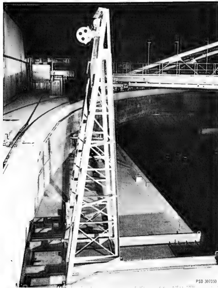
Figure 3 – Leaning Tower (Located at West End of the Basin)
