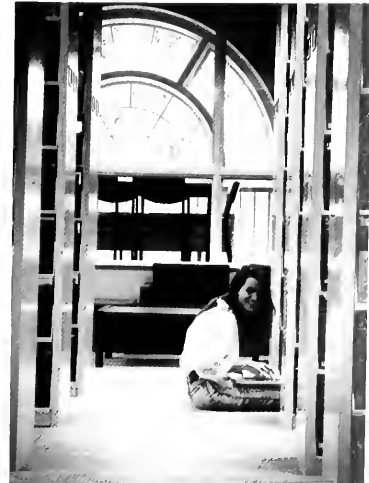
The renovations provide increased space for students. More than 500 students can be accommodated at any one time.
