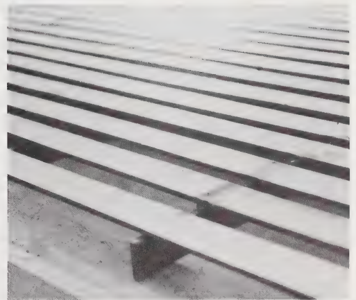
Figure 14 - Homemade slats made of flat iron
