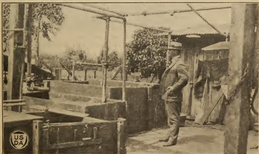
FIG. 20.—Kemoo farm. Concrete vats for steaming garbage.
