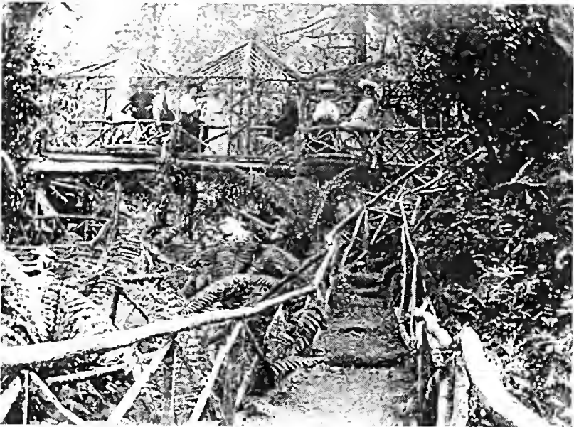
Figure 2. The bridge at the Clematis and Falls hut exemplifies a certain elegance in late 19th Century design.
