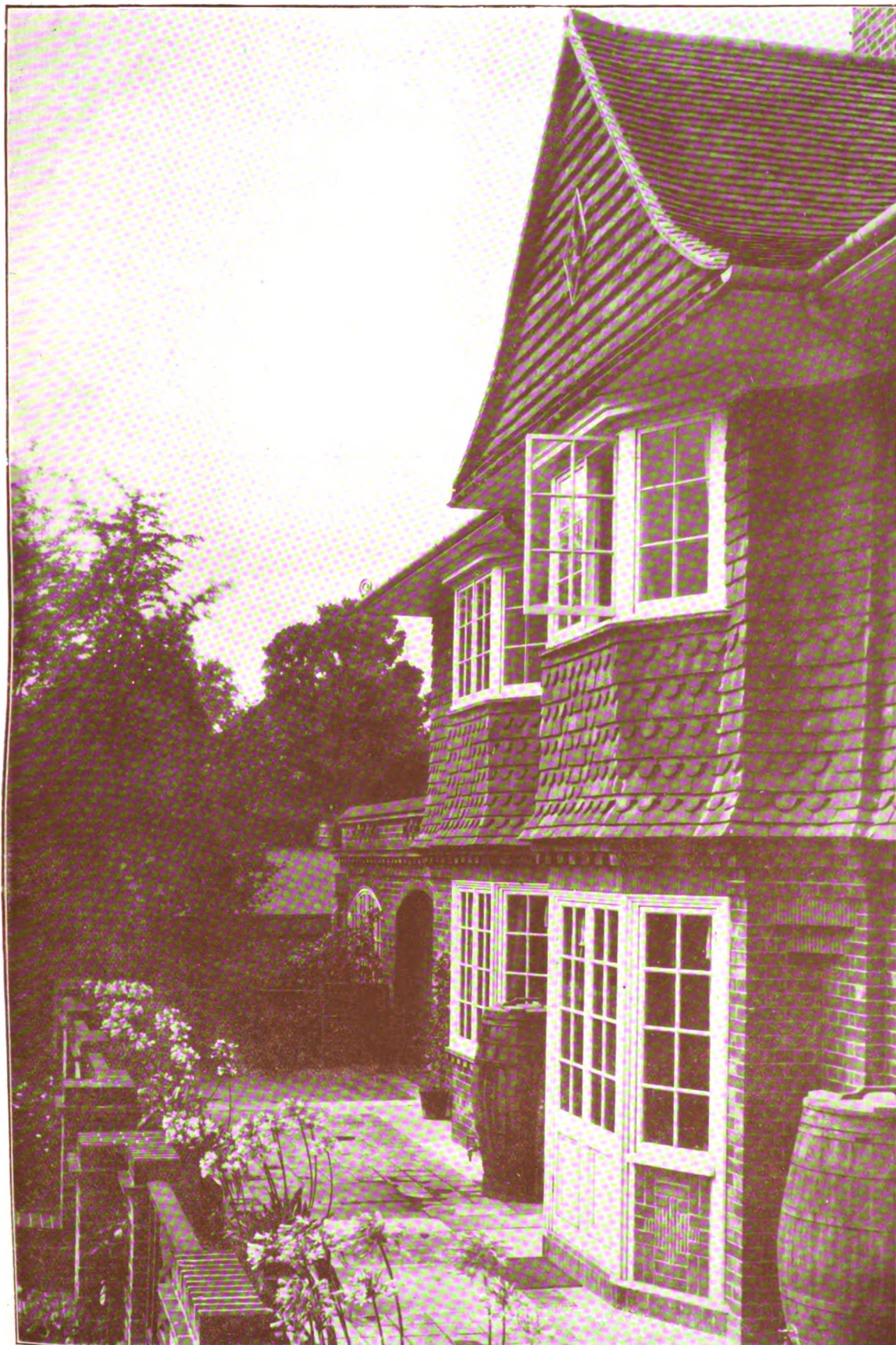
NEW HOUSE, TOTTERIDGE, HERTS : TERRACE AND BAYS. Messrs. H. V. ASHLEY and F. WINTON NEWMAN, FF.R.I.B.A., Architects.
