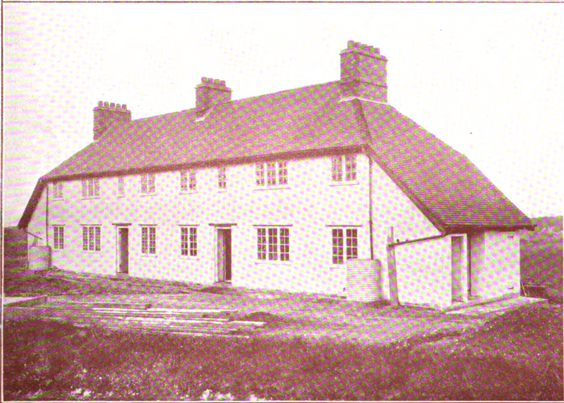
PISE-DE-TERRE COTTAGES, AMESBURY FARM SETTLEMENT.
