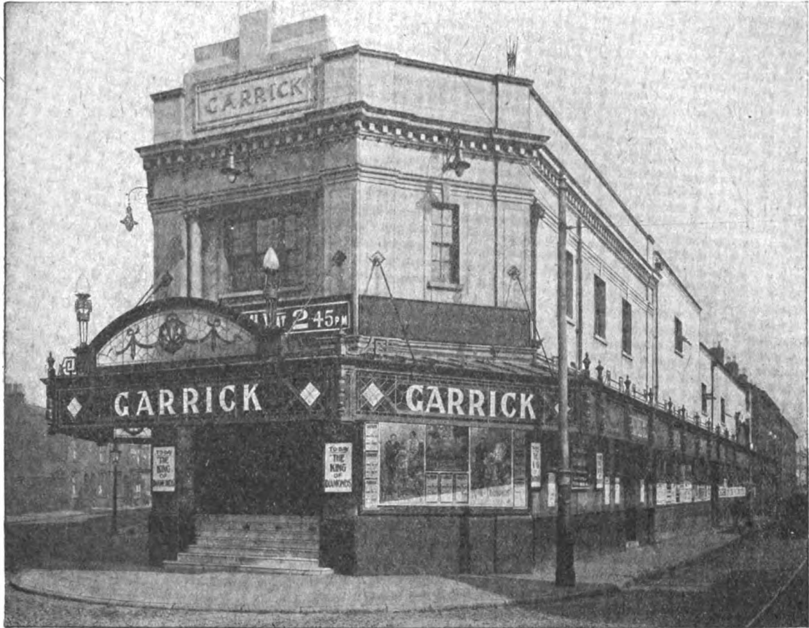
Garrick Picture House, Liverpool, showing Carron Structural Ironwork.
