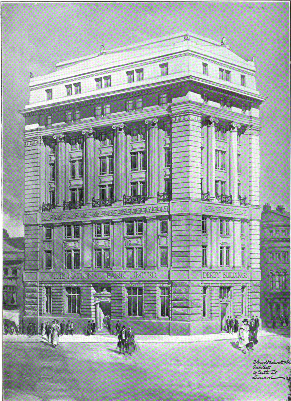
THE NATIONAL BANK, JAMES STREET, LIVERPOOL. Messrs. T. ARNOLD ASHWORTH & SON, ARCHITECTS.
