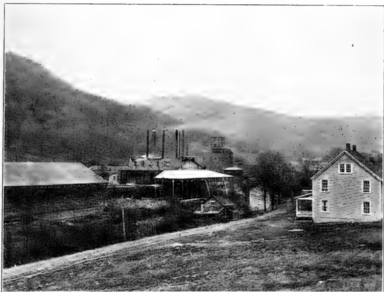
General view of Keery Chemical Co.'s wood distillation plant near Cadosia, N. Y. On the left is the charcoal house; next are the two sets of cooling ovens, and in the center is the oven house with the smokestacks. This plant has a refinery. It is shown on the immediate right of the oven house.
