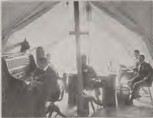
NO. 2—THIRTY-LINE SUBSTATION PATROL BOARD.
