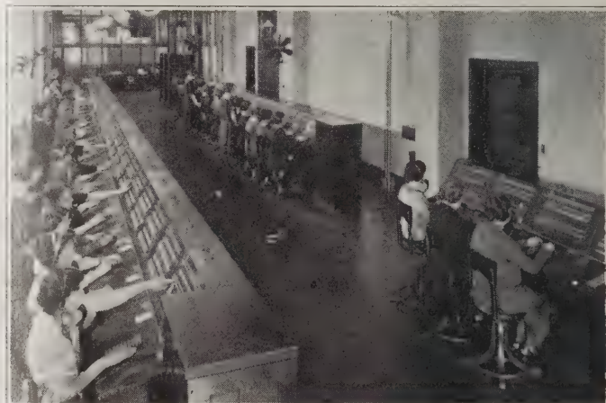
Cordless "B" Switchboard—"Central" on the Left, "State" on the Right.
