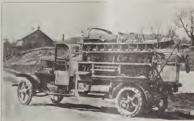
Fig. 12. Latest Type Two-Ton Heavy Construction Unit Showing Tool, Material and Locker Compartments Open.
