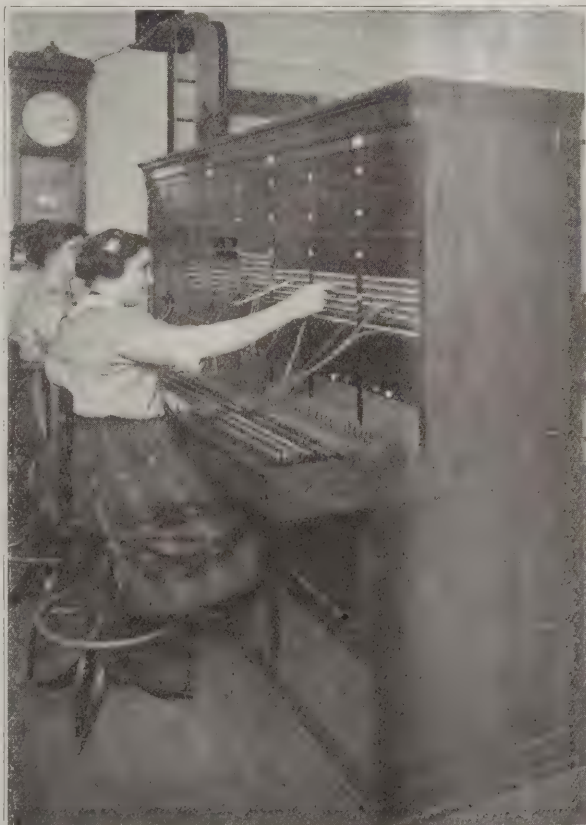
This Modern Switchboard Is Part of the New Equipment Which Enabled the Dan River Company to Give Such Good Service That Its Rates Were Raised.
