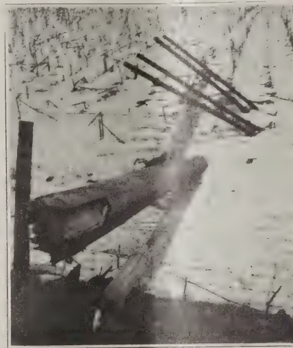
When Telephone and Telegraph Leads Go Down Like This Western Union Lead in Iowa, Line and Maintenance Crews Face Busy Times.—Note Emergency Lead Laid on Ground.
