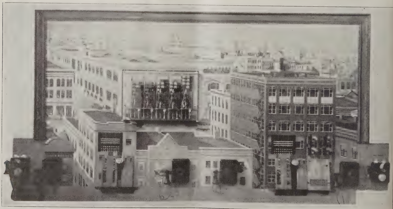
Demonstration Equipment Designed to Give Operators a Knowledge of What Actually Takes Place in Manual-Automatic Cross-Overs.
