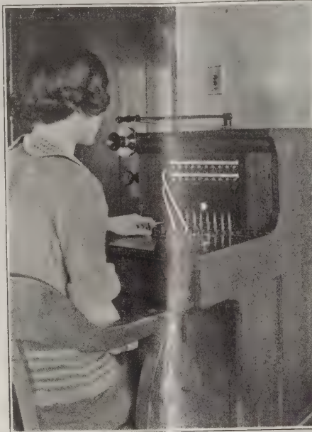
Close-Up of the No. 101-B, P. B. X. Stromberg-Carlson Board in the Temple in Joplin, Mo.
