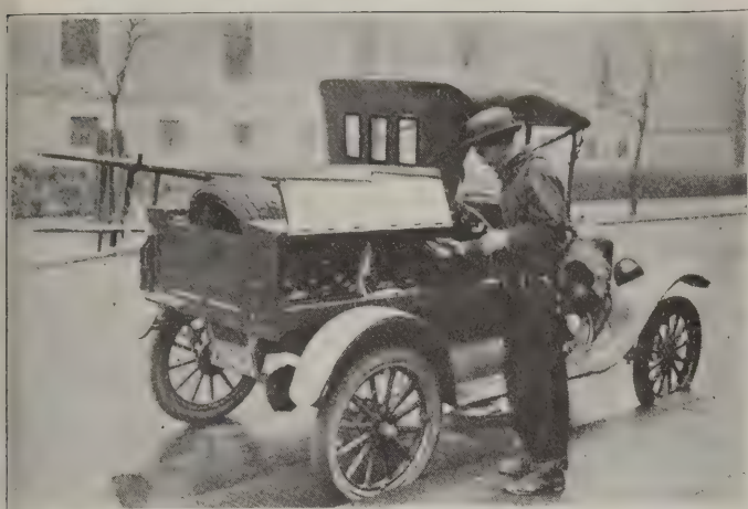
Fig. 8. Ford Runabout of the Latest Type in Telephone Installation Service.
