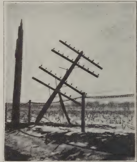
When Telephone and Telegraph Leads Go Down Like This Western Union Lead in Iowa, Line and Maintenance Crews Face Busy Times.—Note Emergency Lead Laid on Ground.
