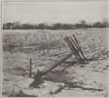
When Telephone and Telegraph Leads Go Down Like This Western Union Lead in Iowa, Line and Maintenance Crews Face Busy Times.—Note Emergency Lead Laid on Ground.
