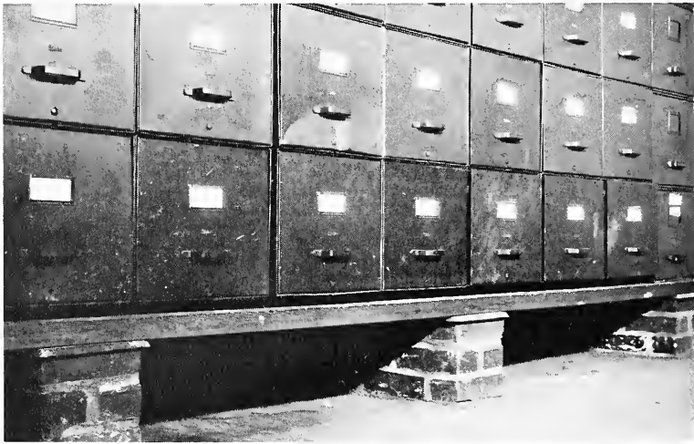
Figure 6. Records stored on a termite-proof rack in the basement of an infested building.
