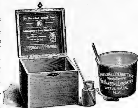
FIG. 49. The Marschall rennet test.
