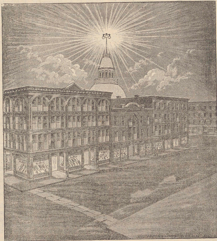
STREET LIGHTING AT WABASH—OLD SYSTEM.
