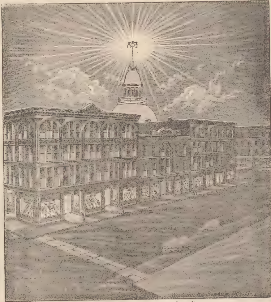
STREET LIGHTING AT WABASH—OLD SYSTEM.
