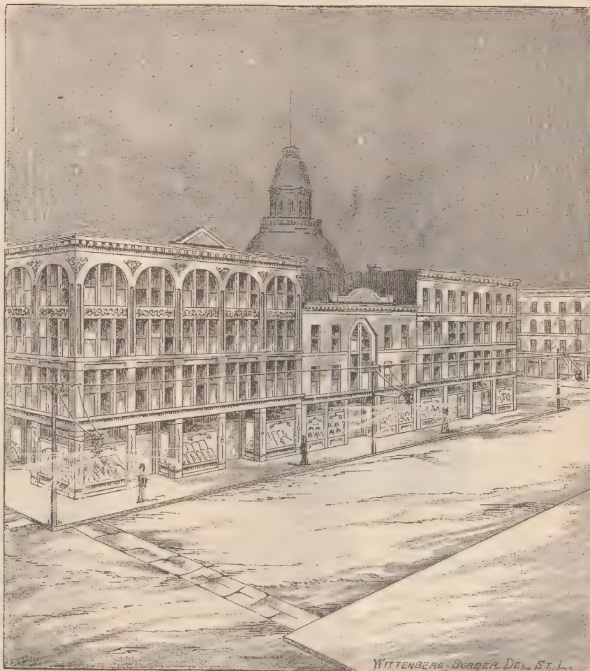
STREET LIGHTING AT WABASH—HEISLER NEW SYSTEM.
