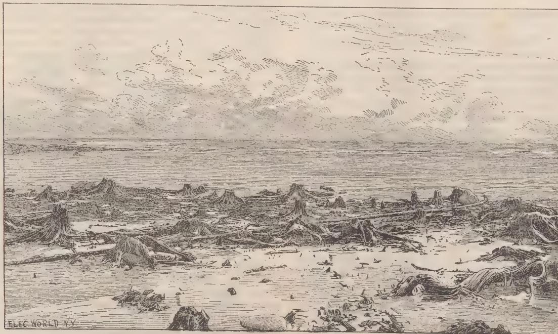
FIG. 1. CABLE LANDING AT RYE BEACH, N. H.
