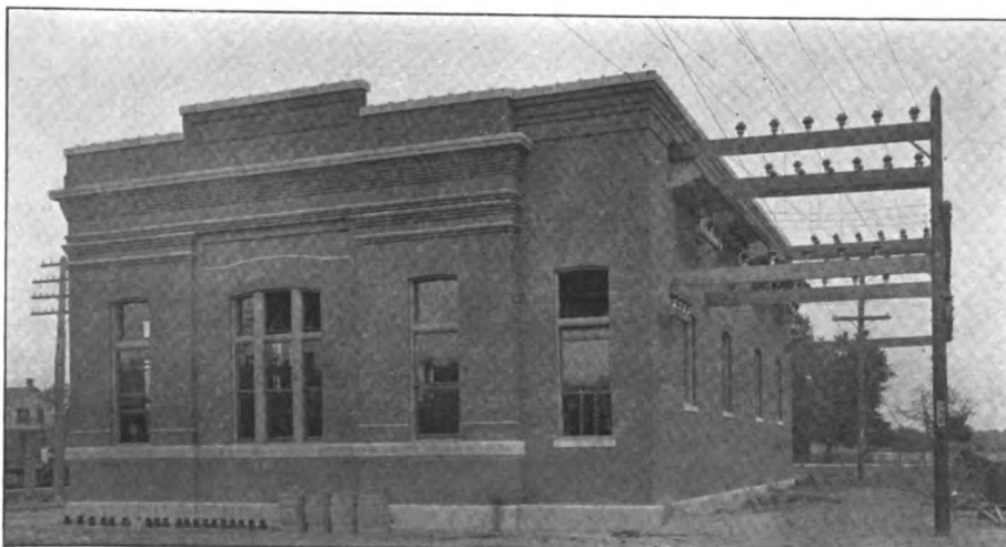
FIG. 10.—EXTERIOR OF THE SUB-STATION AT GLASSBORO
