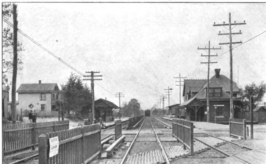
FIG. 2.—THE STATION AT WESTVILLE, SHOWING CATTLE GUARDS, JUMPER BOXES, AND THIRD-RAIL COVERING
