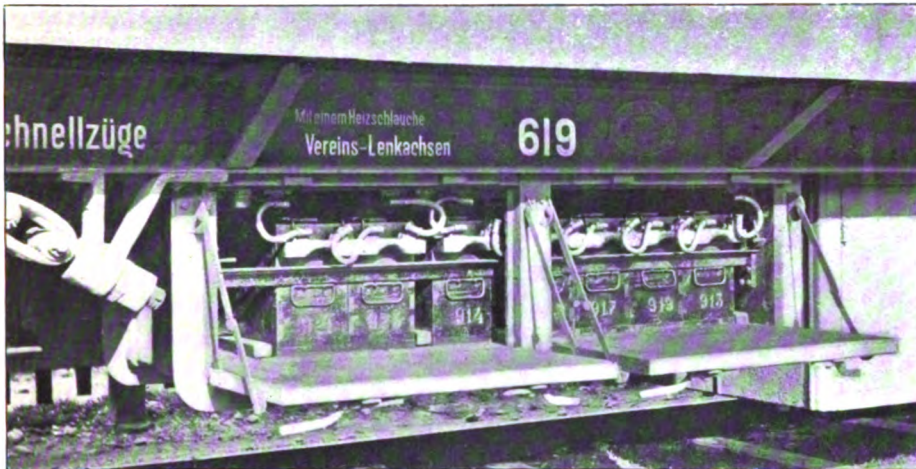
FIG. 1.—BATTERY TRAYS IN PLACE ON AN AUSTRIAN POSTAL CAR
