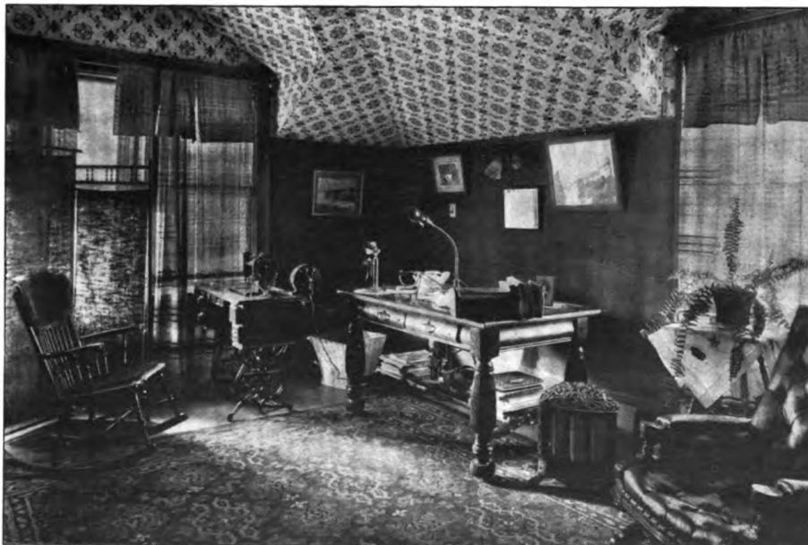
IN THE SEWING-ROOM, THE MACHINE IS RUN BY AN ELECTRIC MOTOR, AND AN ELECTRIC PRESSING IRON IS A CONVENIENT DEVICE
