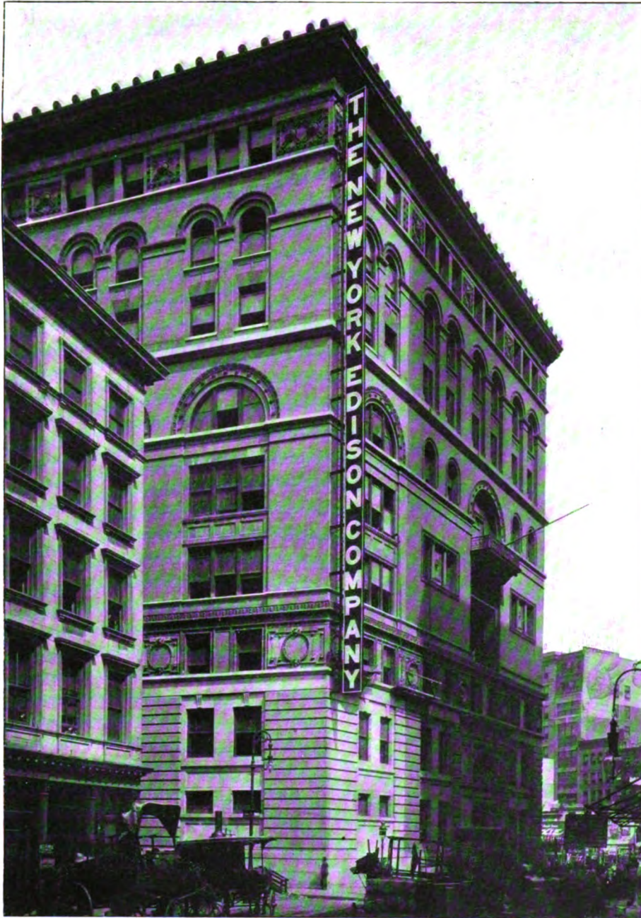
THE LARGEST VERTICAL SIGN IN THE WORLD. IT IS 100 FEET LONG, AND WAS BUILT BY THE METROPOLITAN ENGINEERING COMPANY, OF BROOKLYN, FOR THE DUANE STREET STATION OF THE NEW YORK EDISON COMPANY
