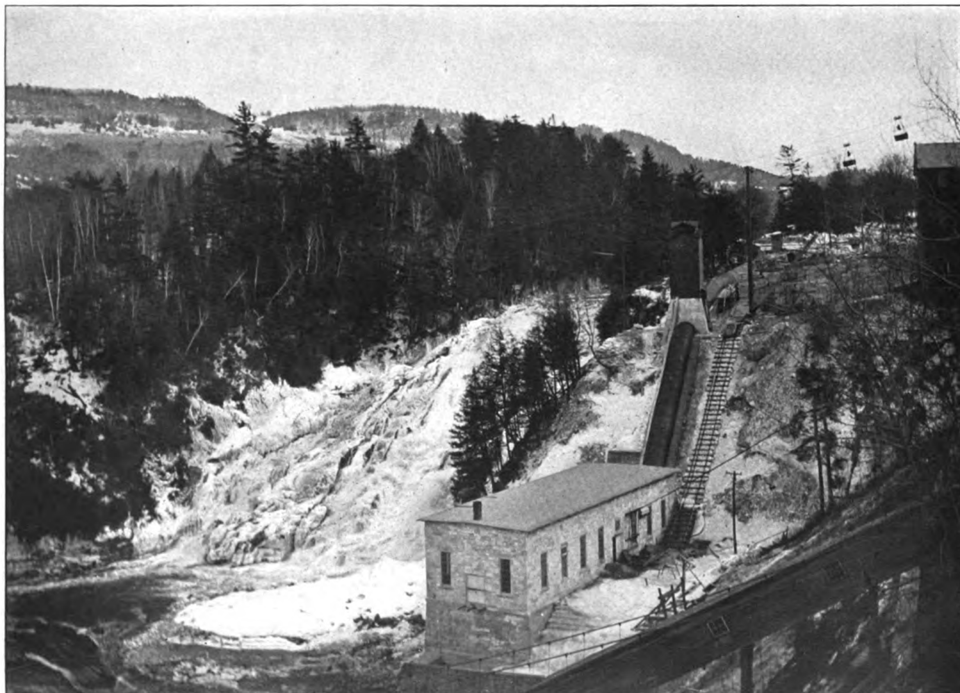
FIG. 1.—GENERAL VIEW OF THE POWER PLANT OF THE VERMONT MARBLE COMPANY, SHOWING THE SUTHERLAND FALLS IN OTTER CREEK
