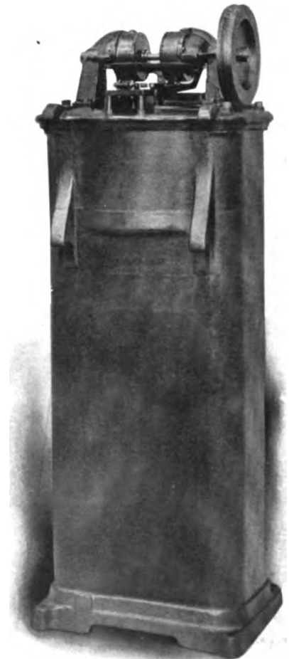
FIG. 5.—AN AUTOMATIC FEEDER REGULATOR
