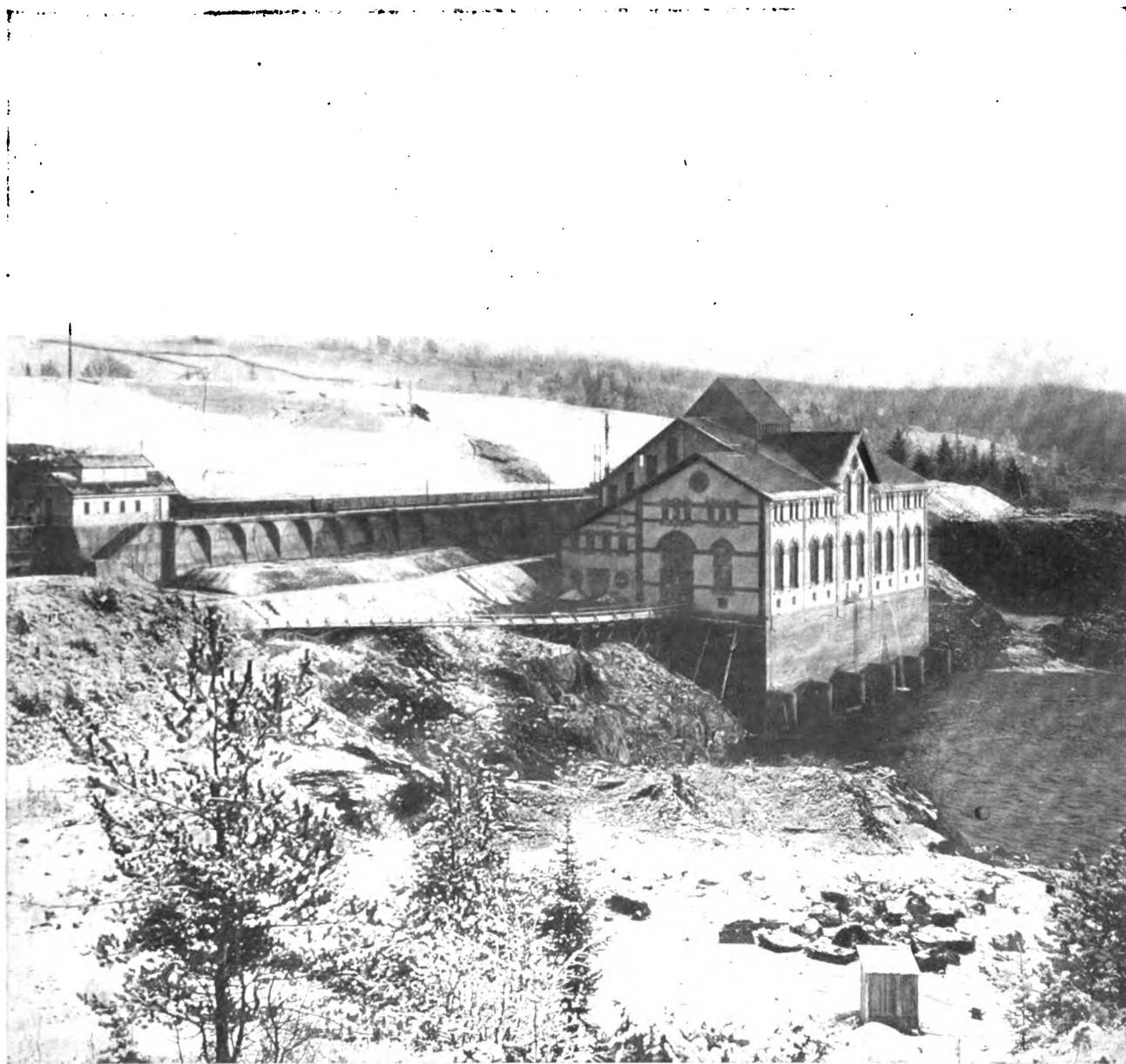
A HYDRO-ELECTRIC POWER PLANT ON THE GLOMMEN RIVER, IN SOUTHEASTERN NORWAY. SEE PAGE 247
