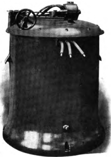
FIG. 17.—A THREE-PHASE REGULATOR
