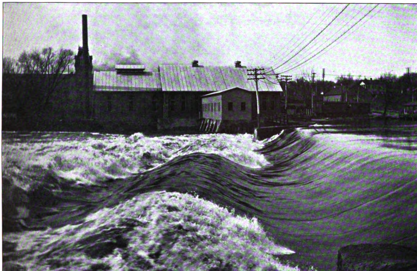
FIG. 5.—THE UPPER DAM AND CENTRAL PLANT OF THE JANESVILLE ELECTRIC COMPANY AFTER COMPLETION
