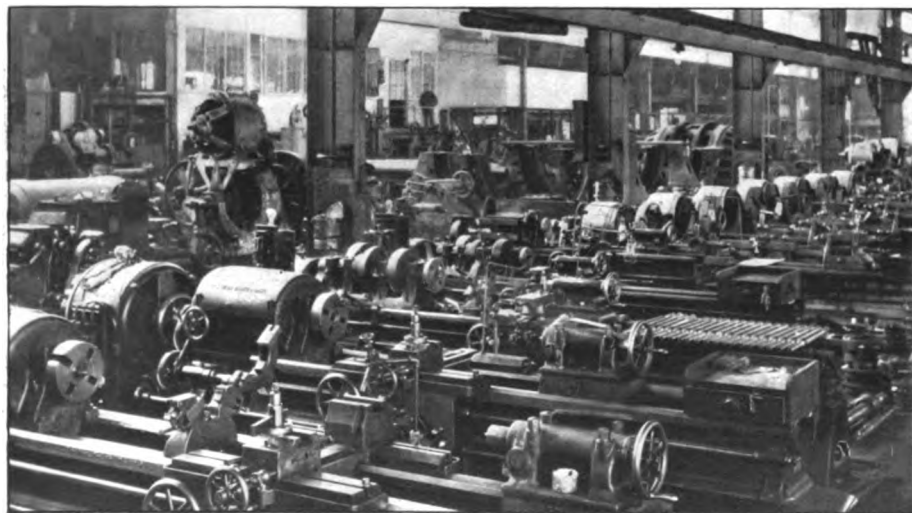
INTERIOR OF ALLIS-CHALMERS' MACHINE SHOP NO. 1, SHOWING MOTOR-DRIVEN LATHES
