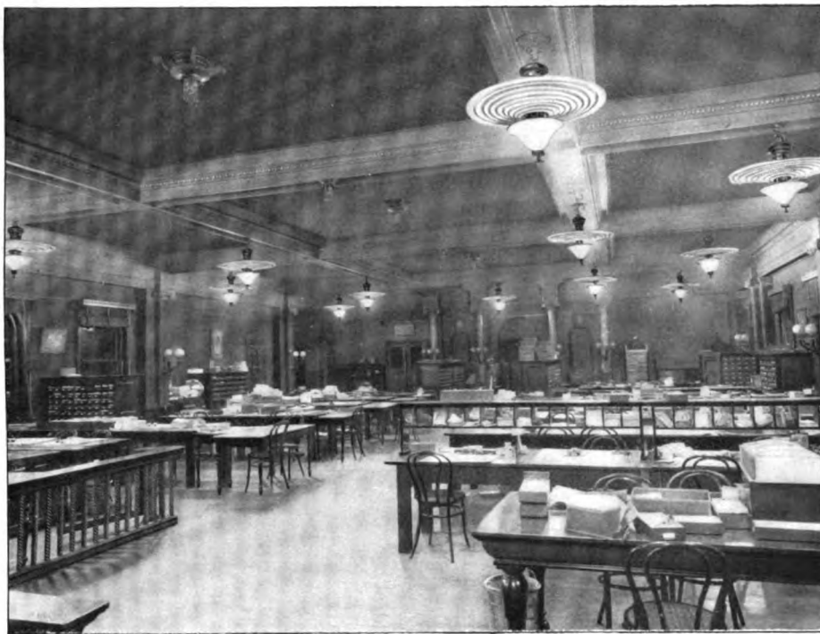
ARC LAMPS WITH CONCENTRIC DIFFUSERS FOR OFFICE LIGHTING
