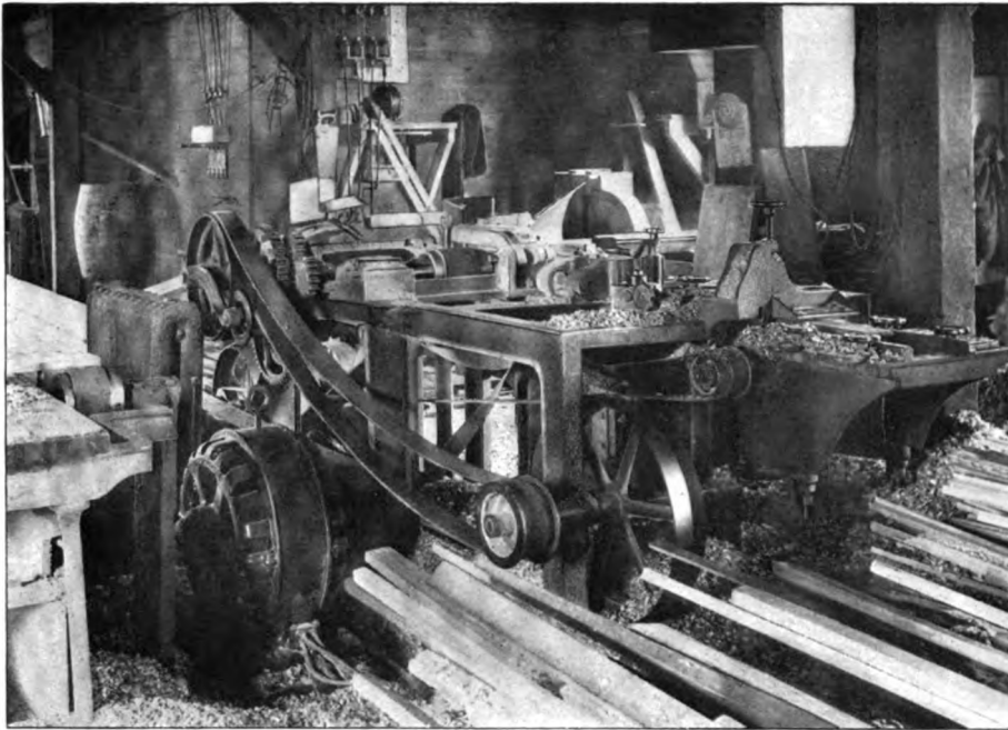
A MOULDING MACHINE DRIVEN BY A 15-H. P. WESTINGHOUSE INDUCTION MOTOR IN THE EGGERS & GRAHAM LUMBER MILL
