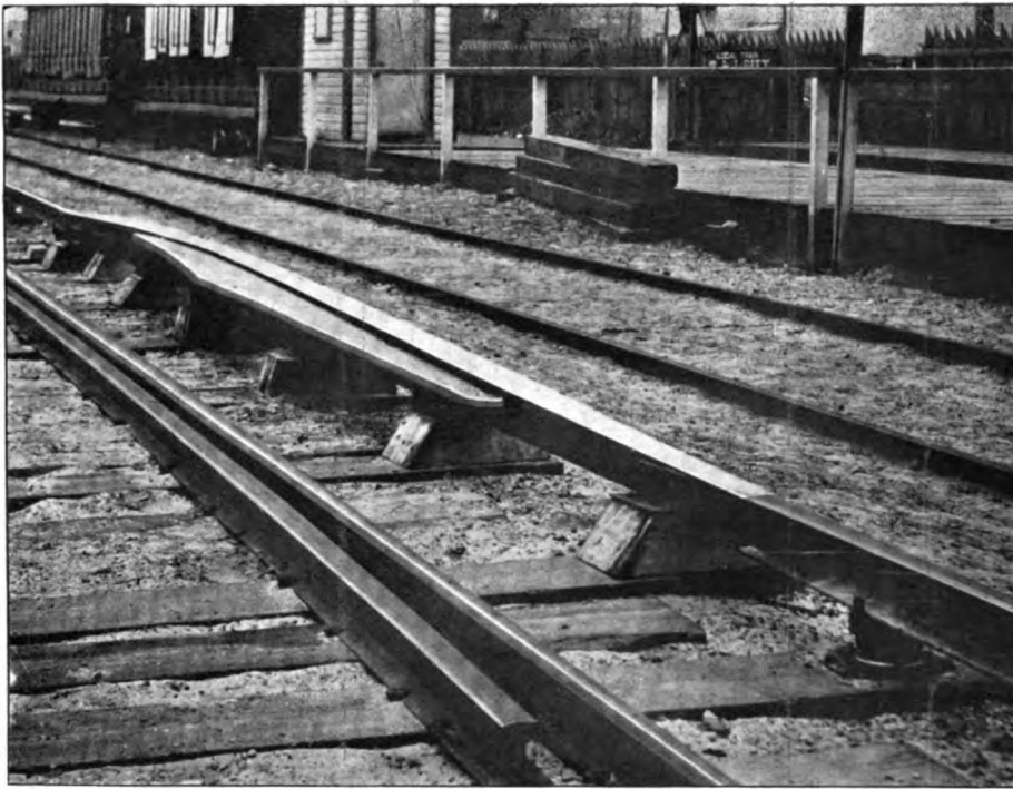
FIG. 6.—A CAM IN THE THIRD RAIL FOR CHANGING THE POSITION OF THE SHOE
