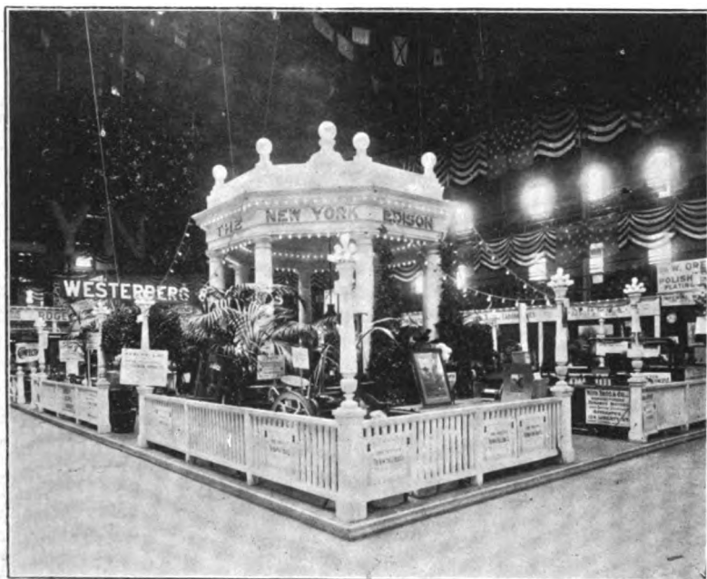
EXHIBIT OF THE NEW YORK EDISON COMPANY.
