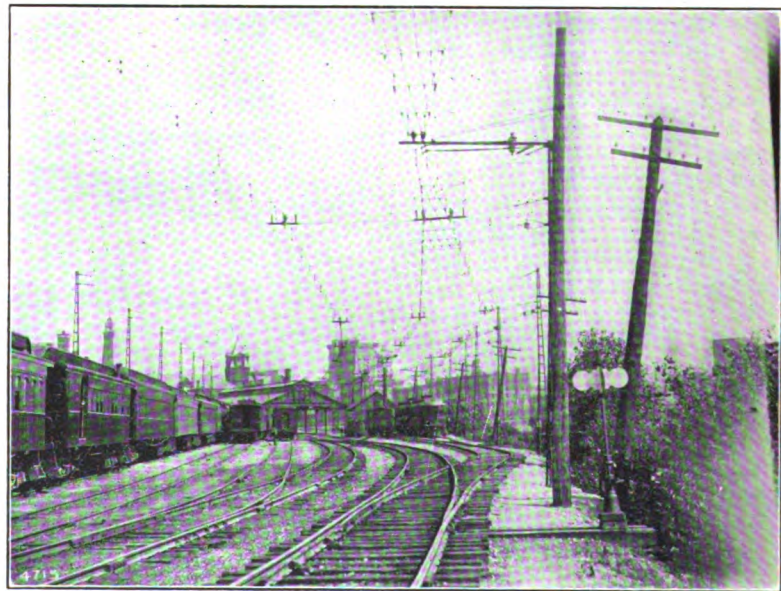
ROCHESTER TERMINAL YARD—OVERHEAD CONSTRUCTION—FOUR ELECTRIFIED TRACKS.
