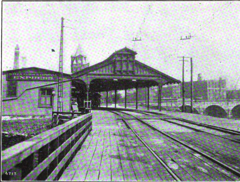
PASSENGER TRAIN SHED—ROCHESTER TERMINAL—SHOWING OVERHEAD CONSTRUCTION.
