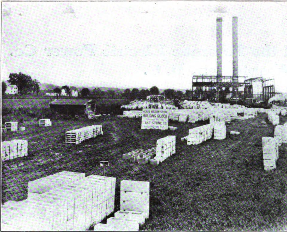
THE STATION AT BENNINGS IN COURSE OF ERECTION
