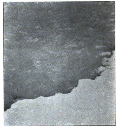
FIG. 3.—SLUSH PACKED IN FRONT OF RACKING
