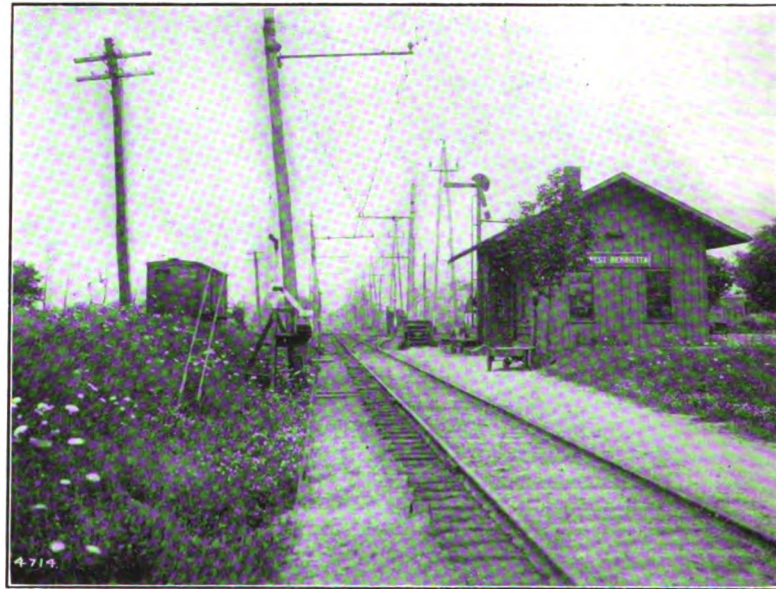
OVERHEAD BRACKET CONSTRUCTION—MAIN LINE AND SIDING AT WEST HENRIETTA STATION.
