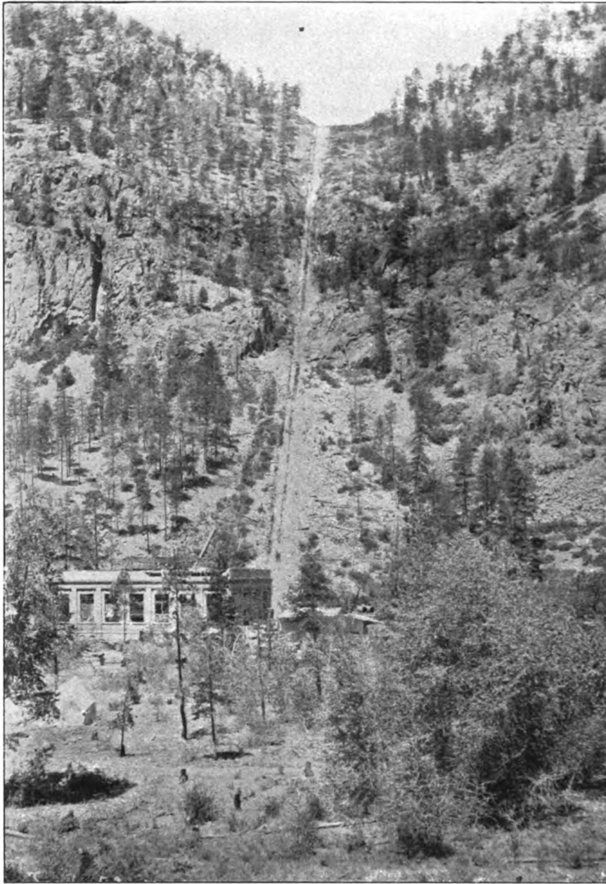
FIG. 5.—THE POWER HOUSE AND PART OF THE PIPE LINE
