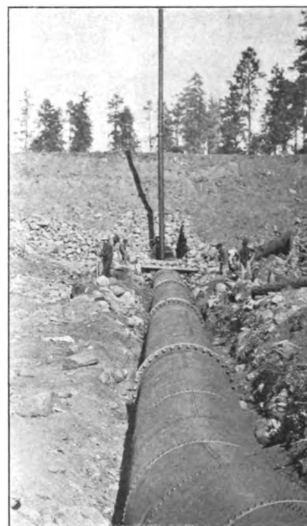
FIG. 10.—A PART OF THE FOREBAY DAM, SHOWING THE STANDPIPE
