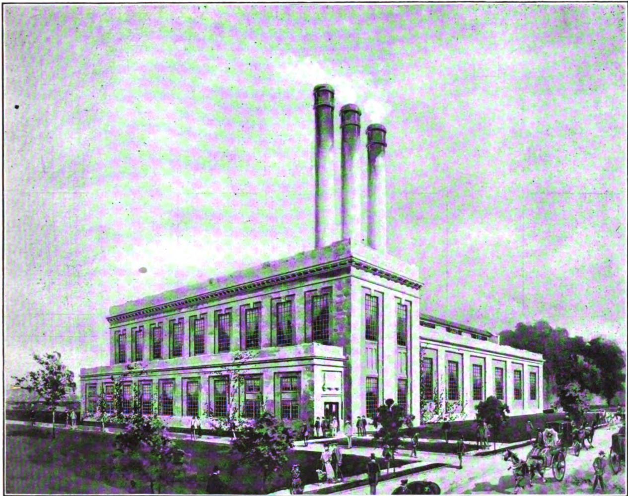
NEW CENTRAL GENERATING STATION OF POTOMAC ELECTRIC POWER COMPANY AT BENNING, D. C.
