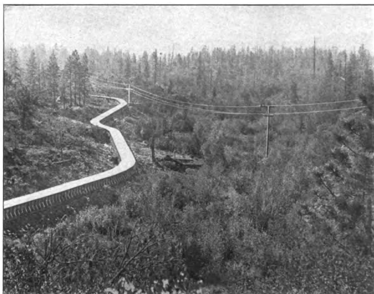
FIG. 8.—PART OF THE FLUME CONNECTING CASCADE RESERVOIR WITH THE FOREBAY. A PART OF THE TRANSMISSION LINE IS ALSO SHOWN
