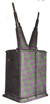
FIG. 22.—88,000 VOLT OIL-IMMERSED CHOKE COIL, WESTINGHOUSE ELEC. & MFG. CO., PITTSBURG, PA.
