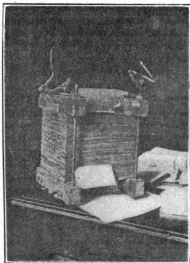
Fig. 2.—STANLEY TRANSFORMER AS BUILT IN 1885
