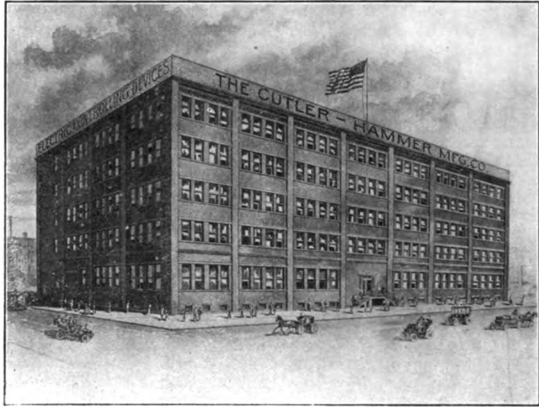
NEW CUTLER-HAMMER FACTORY
