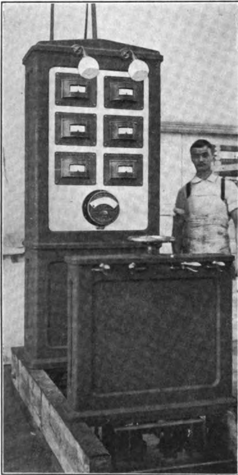
Fig. 11.—AMERICAN (WESTINGHOUSE) CONTROL PEDESTAL AND POST, NIAGARA FALLS POWER COMPANY
