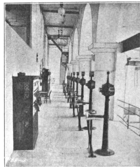
Fig. 4.—CONTROL PEDESTALS IN OPENING GALLERY.
