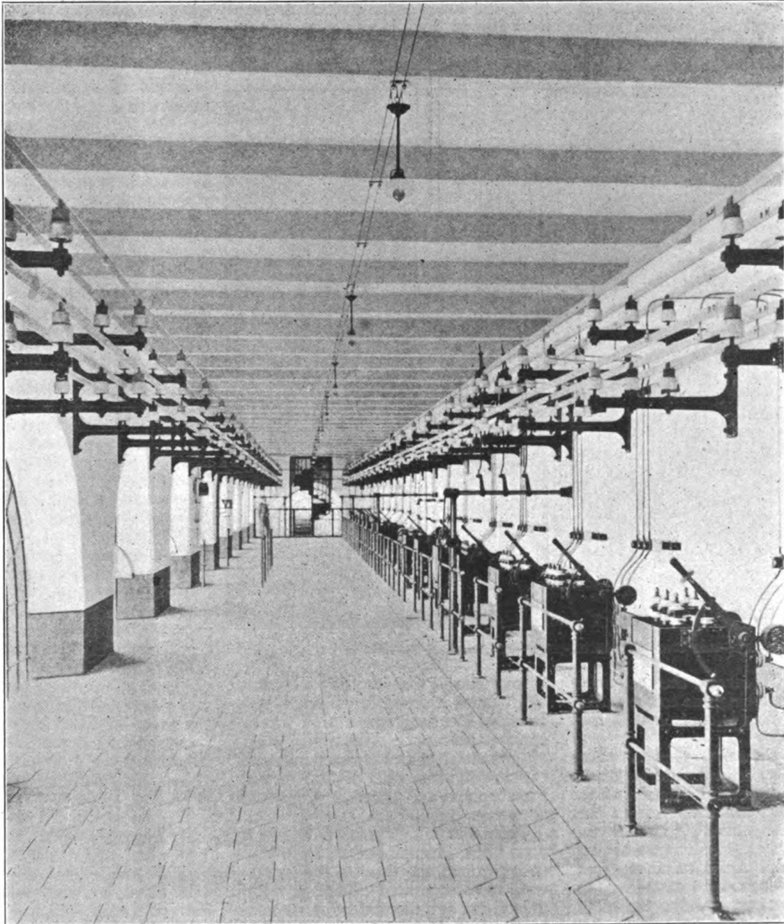
Fig. 20—FEEDER AND BUS-ROOM—HAUTERIVE STATION
