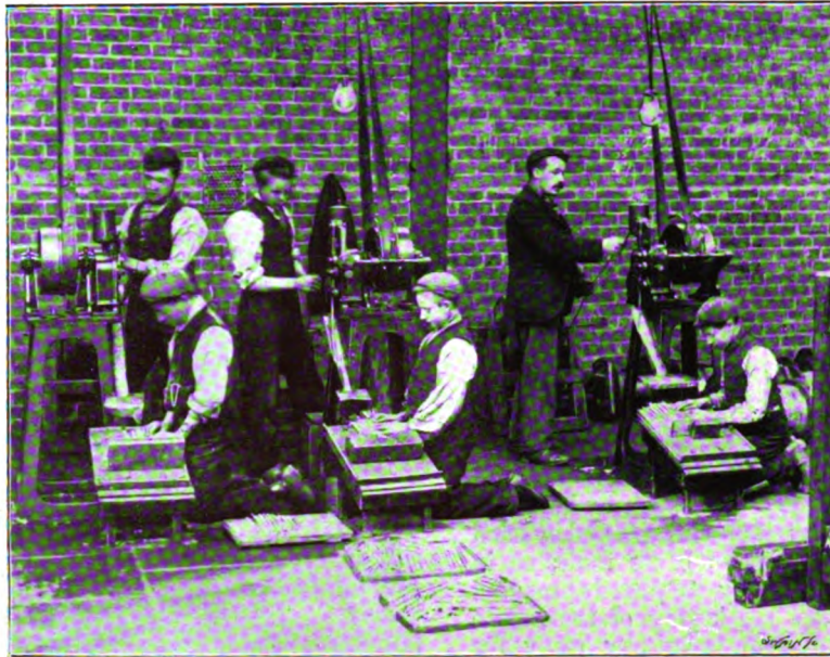
FIG. 7.—THE GIMPING OF THE LEAD STRIP.
