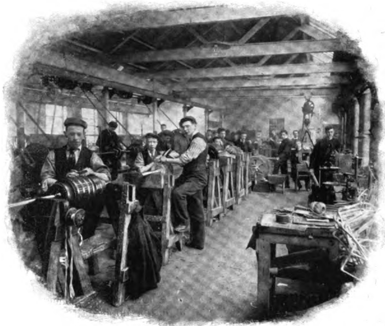
MAVOR & COULSON'S.—ARMATURE WINDING SHOPS.
