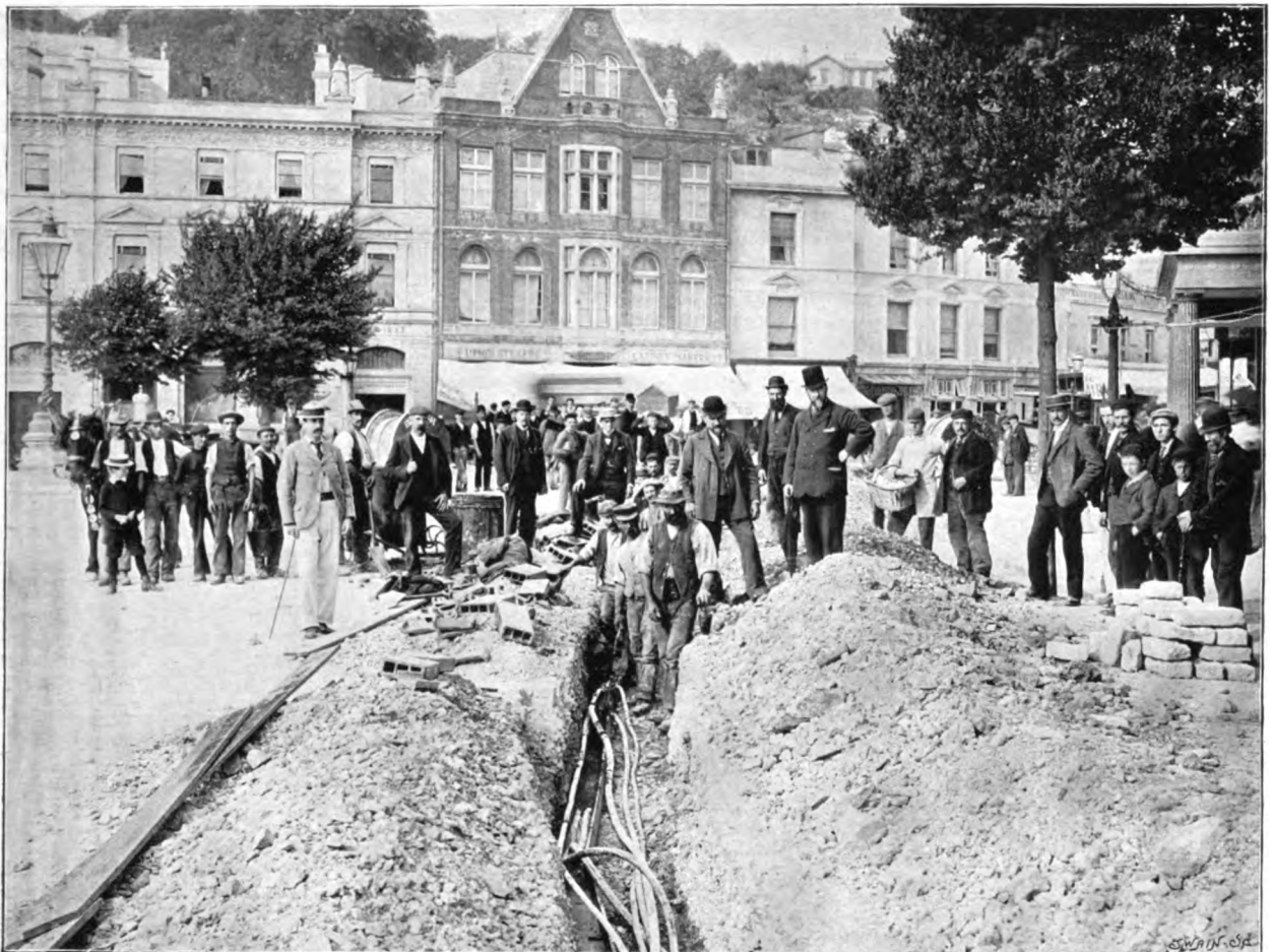
LAYING THE MAINS.
