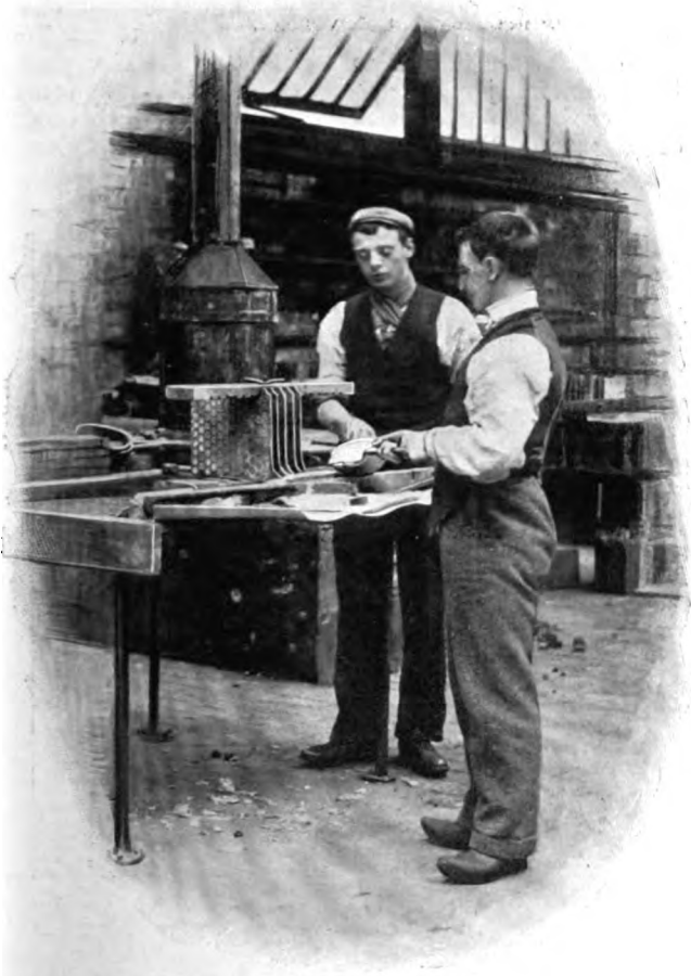
FIG. 5.—CASTING NEGATIVE SECTIONS.
