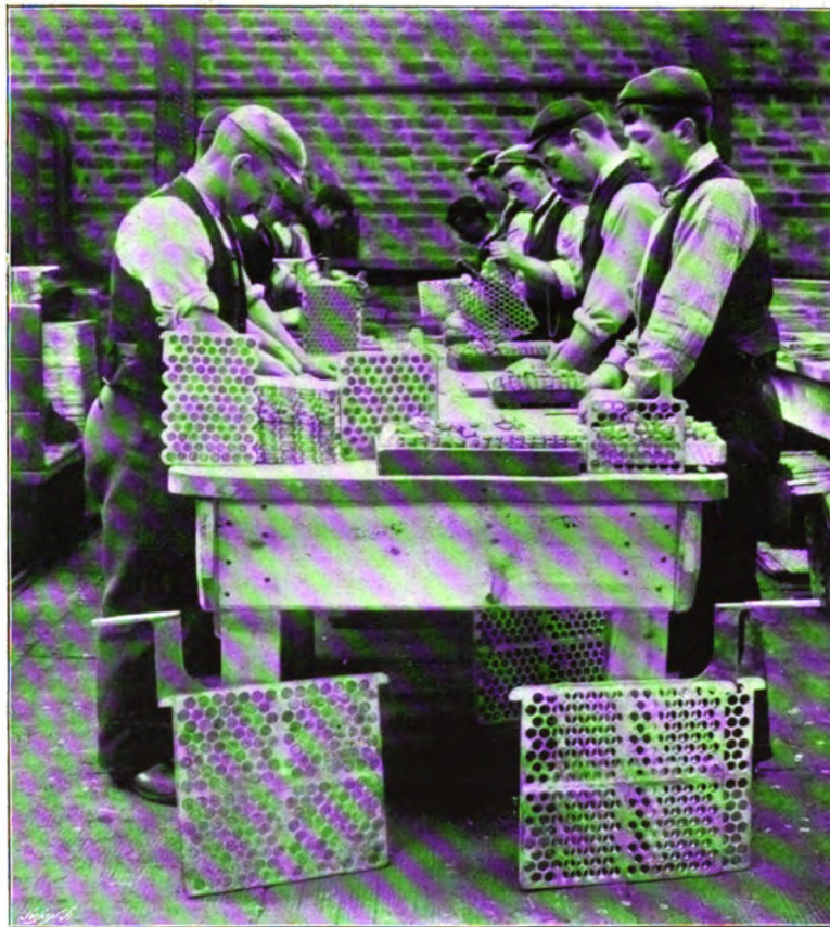
FIG. 9.—PRESSING THE ROSETTES INTO THE POSITIVE GRIDS.
