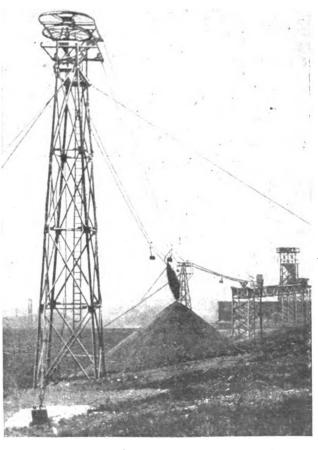
Fig. 3.—RETURN TERMINAL OF ROPEWAY, AND CARRIER DISCHARGING ASHES.
