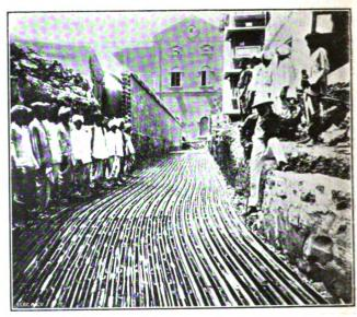
Fig. 22.—Feeder Cables from Receiving Station.
