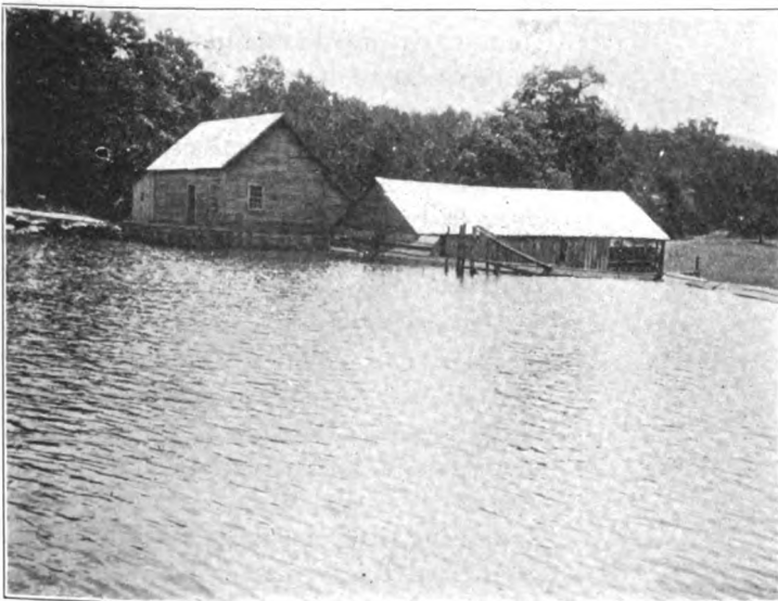
LOOKING TOWARD THE TOP OF THE DAM, AND SHOWING THE BUILDING CONTAINING THE GRIST MILL, SAW MILL AND DYNAMO ROOM.
