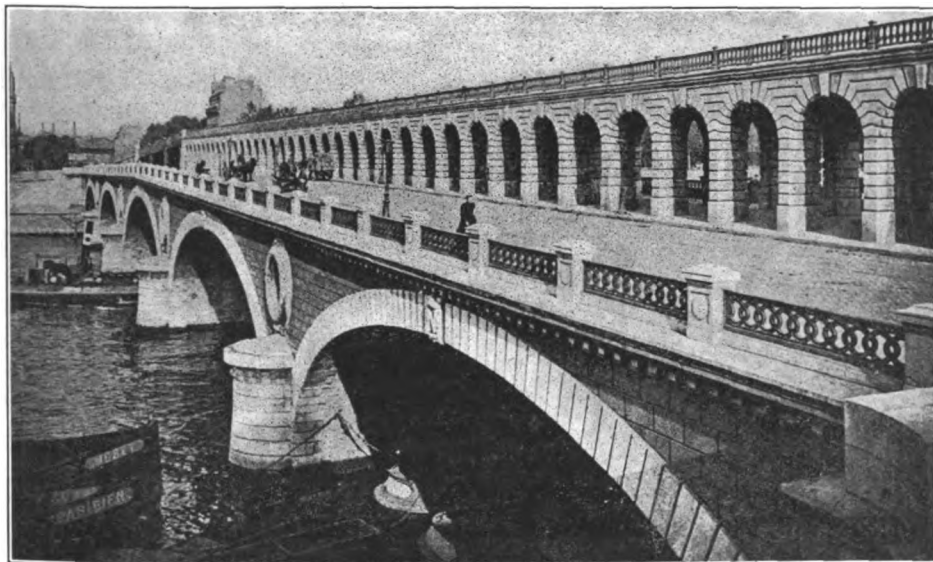
THE BERCY VIADUCT OVER WHICH THE TRACKS OF THE PARIS METROPOLITAN SYSTEM HAVE BEEN LAID.
