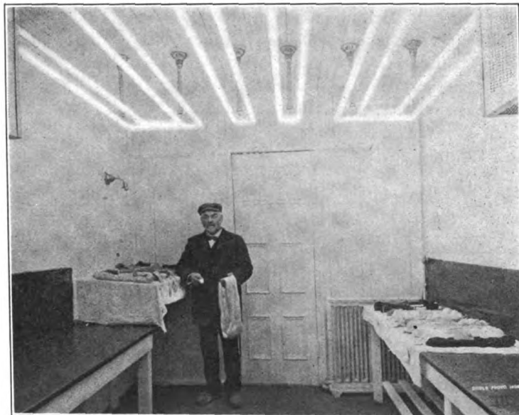
FIG. 3.—MOORE HAIRPIN UNITS IN THE COLOR-MATCHING DEPARTMENT OF THE WEIDMANN SILK MILLS.
