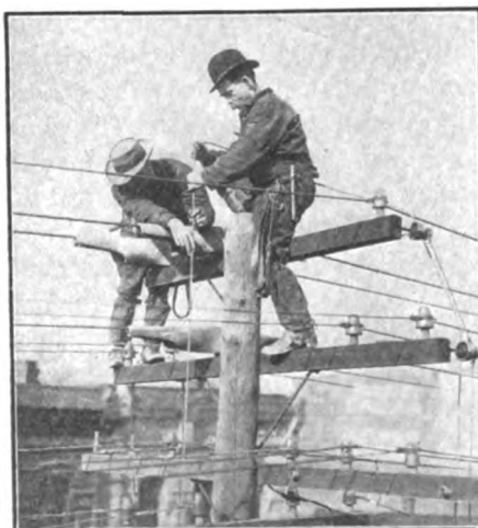
VIEWS SHOWING THE LINEMEN'S PROTECTIVE SHIELD IN USE ON HIGH-TENSION LIVE WIRES.
