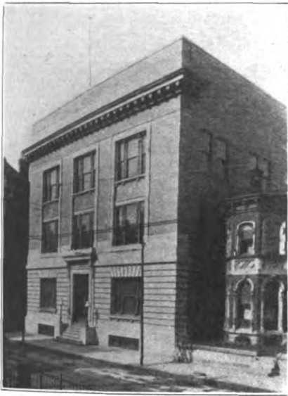
FIG. 1.—NEW WEST EXCHANGE OF THE CINCINNATI & SUBURBAN BELL TELEPHONE COMPANY, CINCINNATI, OHIO.
