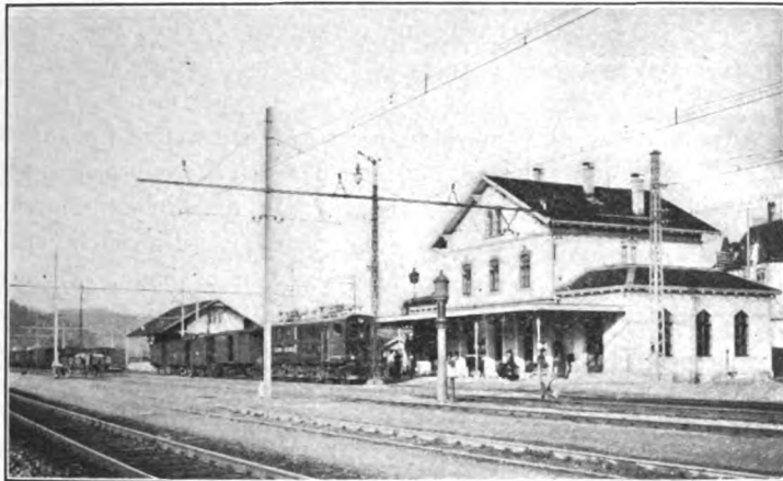
CATENARY SUSPENSION AT RAILROAD STATION AT WETTINGEN; ALSO LOCOMOTIVE NO. 3.
