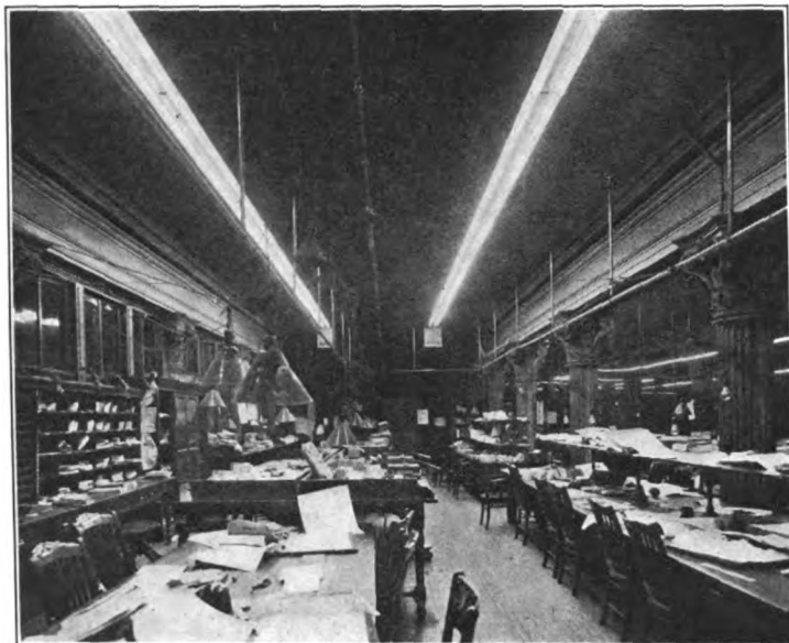
FIG. 1.—MOORE TUBE WITH FRINK REFLECTOR IN REGISTRY DIVISION, NEW YORK CITY POST-OFFICE.
