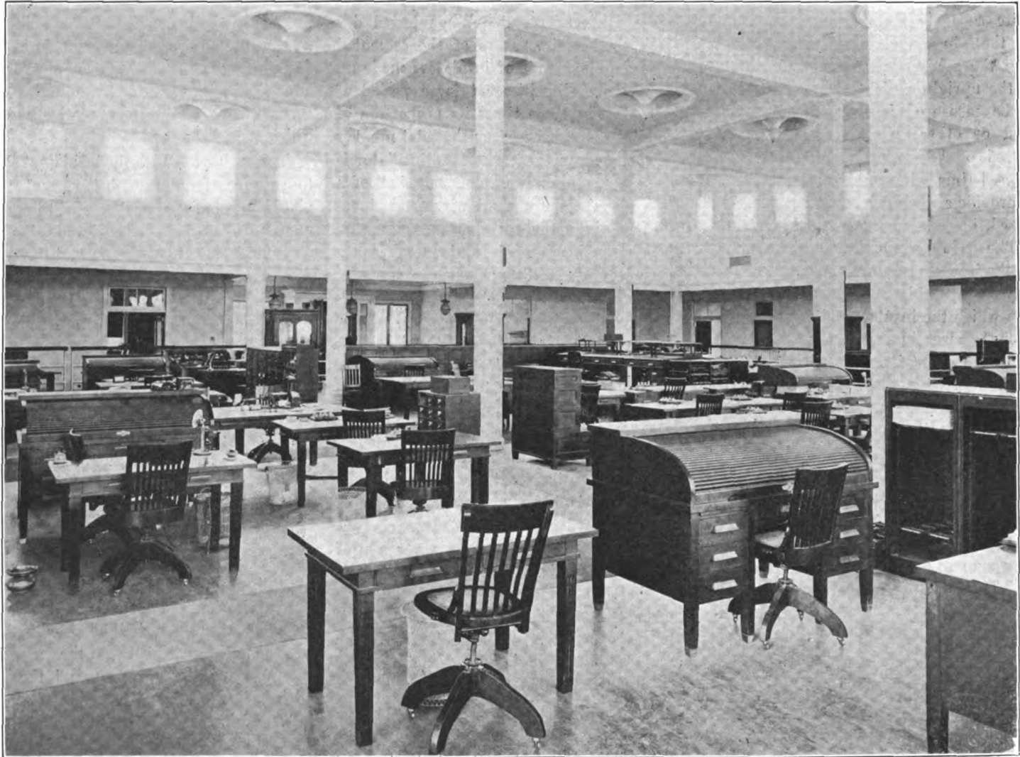
DAYLIGHT PHOTOGRAPH OF THE OFFICE OF THE STANLEY WORKS, NEW BRITAIN, CT.
