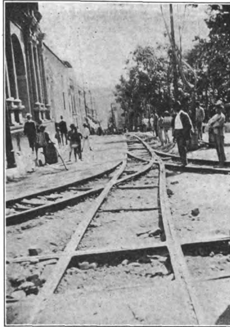
CARACAS TRAMWAYS. SPECIAL WORK, UNDER CONSTRUCTION.
