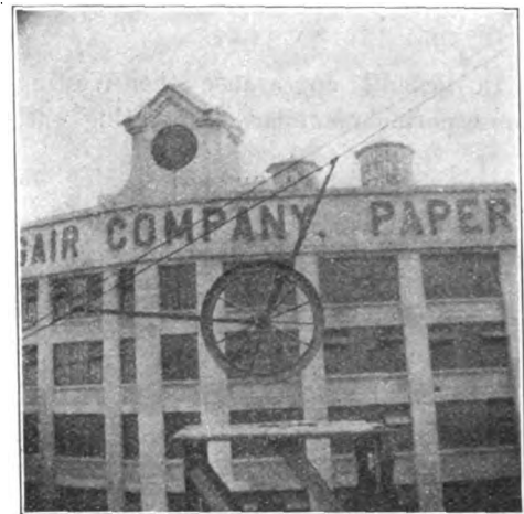
THE HAULING SHEAVE IS ATTACHED BY WROUGHT-IRON LEGS TO A THREE-QUARTERS-INCH TRAVELING CABLE.
