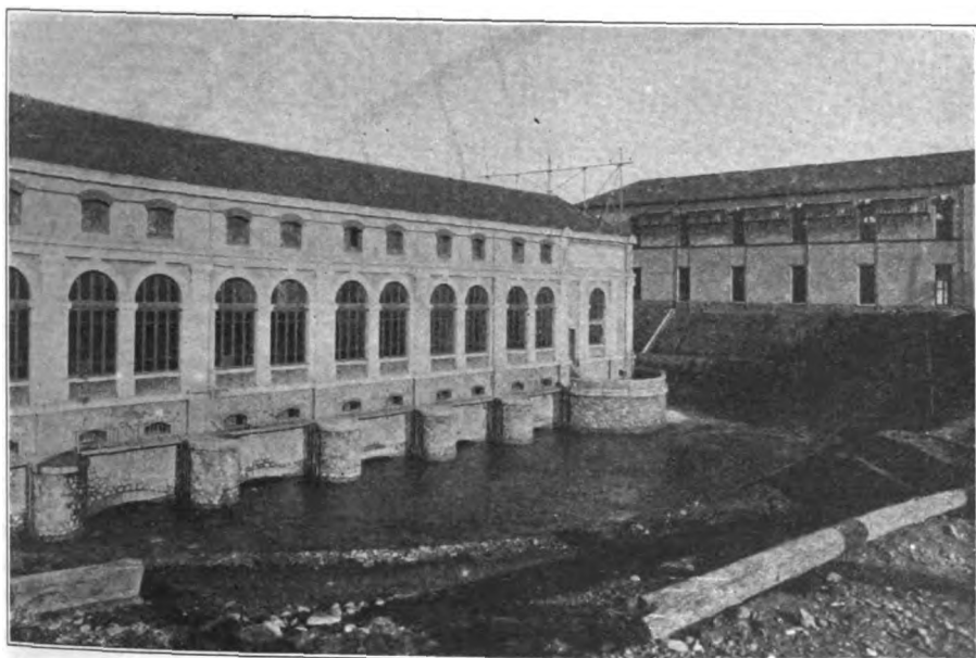
EXTERIOR VIEW OF THE BRILLANNE HYDROELECTRIC PLANT AND TRANSFORMER HOUSE.
