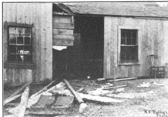
VIEWS SHOWING THE DAMAGE CAUSED BY THE BURSTING OF A RUNAWAY FLYWHEEL.
