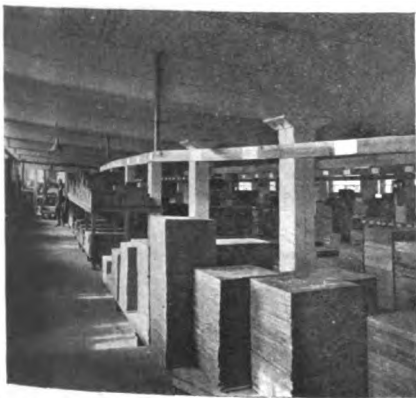
SLATE STORAGE DEPARTMENT OF THE TRUMBULL ELECTRIC MANUFACTURING COMPANY.
