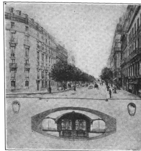
STANDARD FORM OF CONSTRUCTION ON THE NORTH-SOUTH LINE OF THE PARIS METROPOLITAN SUBWAY.
