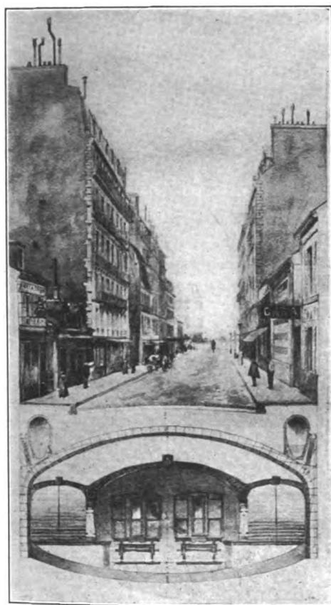
THE FORM OF CONSTRUCTION IN A NARROW STREET—PARIS METROPOLITAN SUBWAY.
