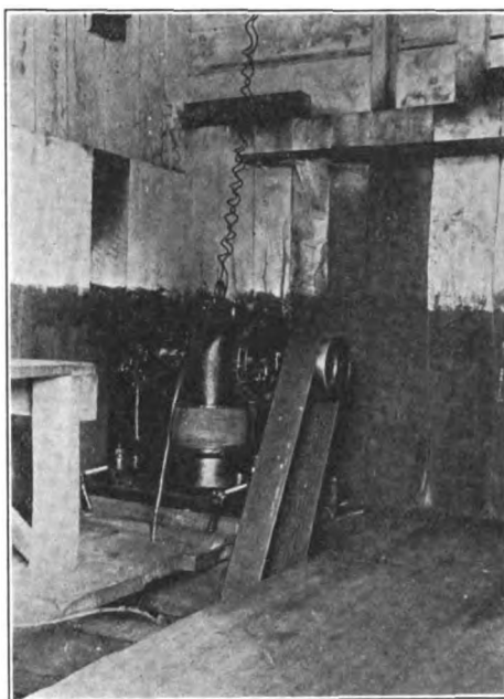
A VIEW OF THE DYNAMO ROOM.
