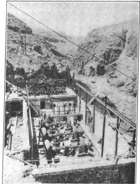
FIG. 2.—HYDROELECTRIC PLANT NEAR AVENTURA, ON RIO LOA, SHOWING METHOD OF CONSTRUCTION.
