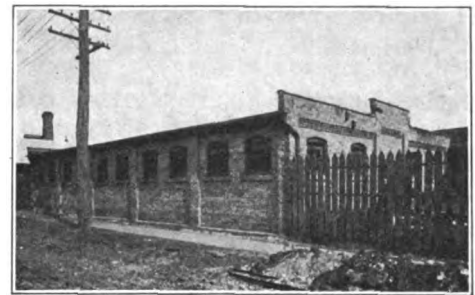
FIG. 4.—BATTERY HOUSE OF THE ELMIRA WATER, LIGHT AND RAILROAD COMPANY, ELMIRA, N. Y.
