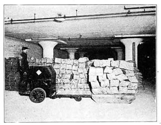
Awkward Loads Like This Are Handled Very Efficiently by Electric Lift-Trucks.
