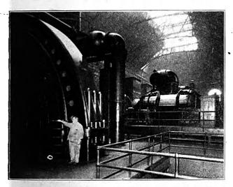
Fig. 2.—Interior of Interborough Rapid Transit Co.'s Power House, Showing Old 7500-hp. Engine-Driven Unit in Foreground and Newly Installed 70,000-kw. Turbine in Rear.
