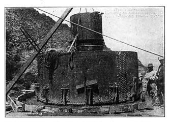
Surge Tank at Pangal Hydroelectric Development, Showing Bottom Steel Section Just After Erection and Anchoring to Concrete Section.
