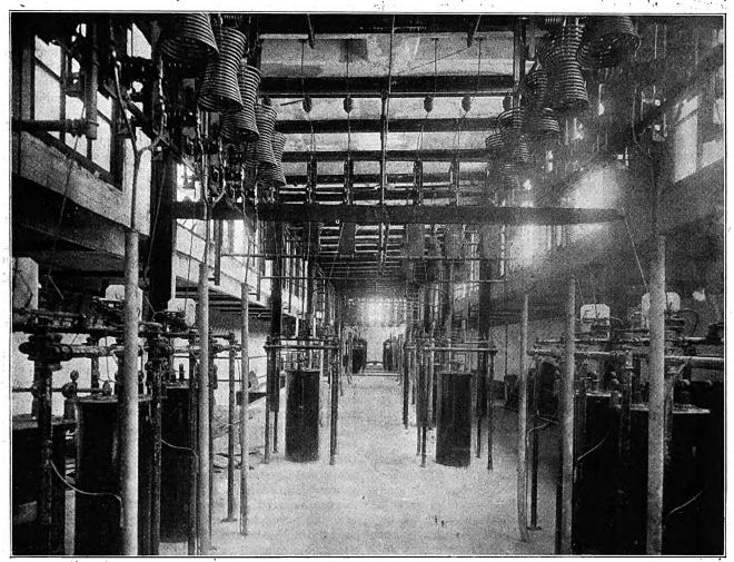
Fig. 4.—Arrangement of Disconnecting Switches and Lightning Protective Apparatus.
