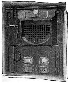
Fig. 5.—Mechanical Soot Blower in Return Tubular Boiler.
