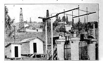
Electrical Apparatus for Dehydrating Crude Oil.
