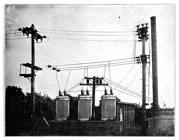
Fig. 1.—Early Type of Pole Structure for 600-Kv-a. Transformers, Transforming from 22,000 to 2300 Volts. Metering on 2300-Volt Side.
