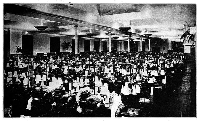
Night View in a Knitting Mill Where Indirect General Lighting Eliminated Complaints About Glare from the Needles and Wiped Out High Labor Turnover.
