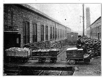
Electric Truck and Trailers Hauling Materials in Foundry.
