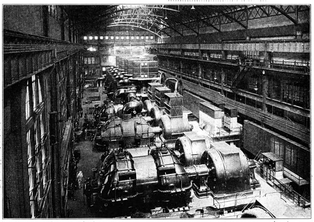
Fig. 1.—General View of Interior of Interborough Rapid Transit Power House, East 74th Street, New York, Showing One of the Westinghouse 30,000-Kw. Cross-Compound Units in Foreground, Newly Installed 70,000-Kw. Triple-Compound Unit In Center and Old 7500-Hp. Engine-Driven Units in Rear.
