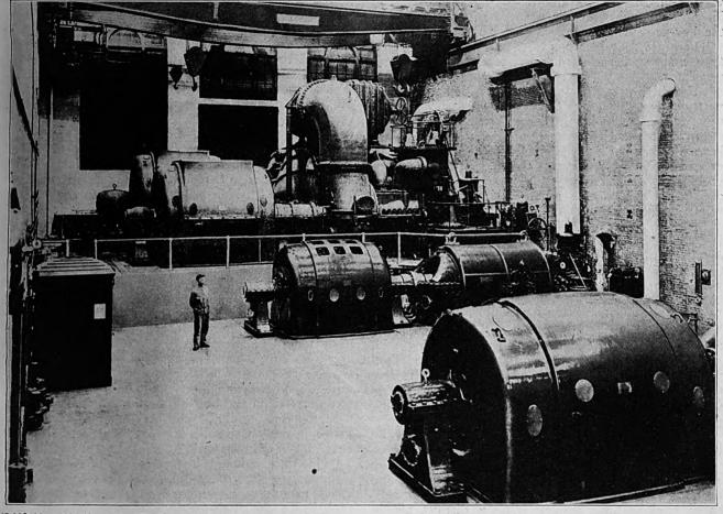
45.000-Kw. Westinghouse Turbogenerator Operating in Station of Narragansett Electric Light Company, at Providence, R. I.
