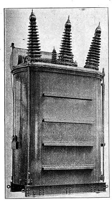
Fig. 1.—High-voltage Side of a Larger Three-phase Transformer With Oil Conservator.
