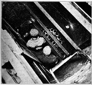
Fig. 6.—View Looking Down Brick Lined Shaft Showing Location of Ducts Ladder and Angle irons.
