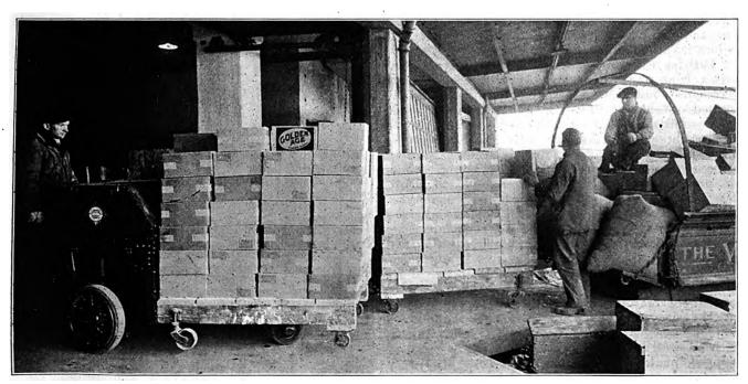
The 9th Street Terminal Warehouse in Cleveland, Ohio, Uses an Electric Lift Truck to Good Advantage in Handling Goods of Ali Kinds.
