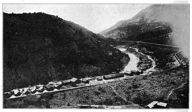
View From Diversion Dam of Rio Pangal Development, Looking Downstream and Showing a Section of the Seven-Mile Pipe Line.
