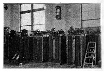
Part of the Bank of 21 Single-Phase, 2300-Volt Regulators on Light and Power Feeders.
