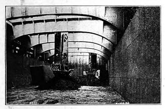
Unloader Leg and Bucket at Work in Hold of a Modern Ore Vessel—Leg Can Rotate in a Circle, Allowing Bucket to Reach Out in All Directions, Taking Out as Much as 97% of Cargo Without Shoveling—Note Position of Bucket Operator Directly Above Bucket.
