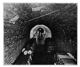
Fig. 3.—Conduit Stacked Ready for Use. Cheesecloth is Used to Prevent Ducts From Being Clogged Up During Assembly.
