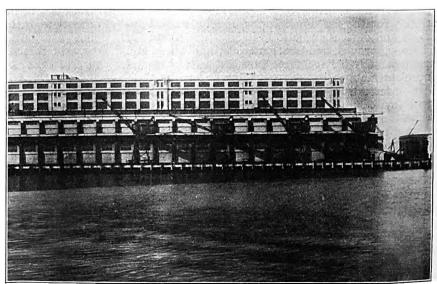
View Taken From Roof of Wharf Shed of Four Semi-Portal Bridge-type Dock Cranes
