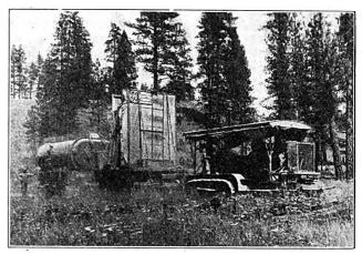
Transformer Element and Tank Being Hauled on 10-ton Trucks by a Holt Caterpillar Tractor.
