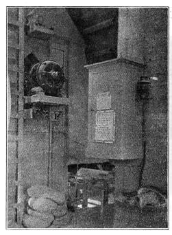
Fig. 4.—71/2-hp. Motor Driving Klinker Elevator.
