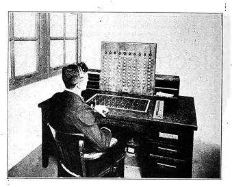
Dispatcher's Desk for "Operatorless" Elevator System. This
