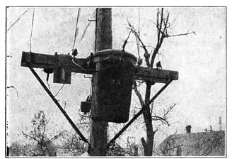
Maximum Demand Meter Installed Upon Pole for Measuring Demand on 25-Kw. Transformer.
