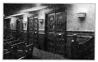
Fig. 2—Wall Urns Serving as Lighting Units at Main Entrance to Auditorium Under Balcony—Ordinary Brackets Would Cause Glare.
