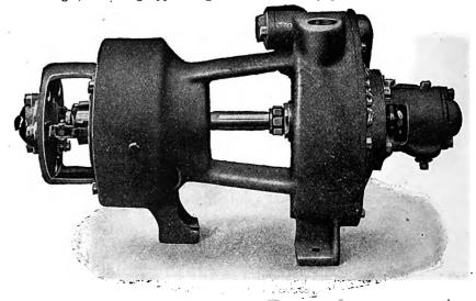
Buda-Ross Steam-Turbine Electric Light Plant of 1 Kw. Capacity.
