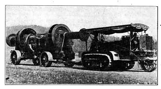
Holt Caterpillar Tractor Pulling 381/2-ton Load Consisting of Turbine Runners and Shaft.
