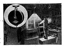
The Anderson "Reelite" consists of a reel unit carrying approved portable reinforced cord. The cord-winder is of the four-spring type insuring long life even under severe usage. The base of the device is designed to attach to any 4-in. outlet box, or direct to the ceiling. To operate it is necessary merely to raise or lower like an ordinary windowshade.
