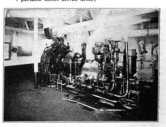
One of Six Turbogenerator Sets for Supplying Lights, Fans, Cranes, Wireless, and Scores of Auxillary Motors.
