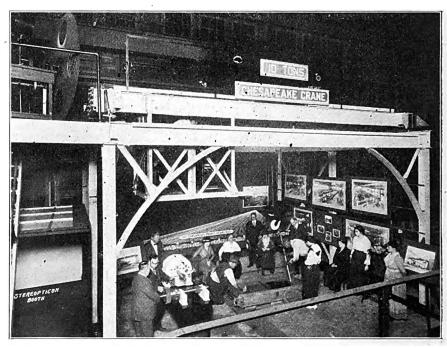
A 10-Ton Chesapeake Electric Traveling Crane Being "Tuned Up" at the Works for Exhibition Before the American Foundrym en's Association.
