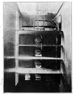
Fig. 5.—Truck Housing Showing Disconnecting Devices and Barriers.
