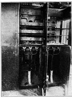
Fig. 6.—Truck Housing, Showing Bus Compartment and Method of Bringing Up Cables.
