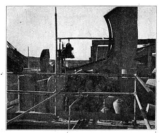
Fig. 3.—1/4-hp., 440-voit., 1725-r.p.m. Westinghouse Single-Phase Motor Driving Slurry Feed Control Dipper.
