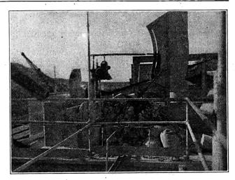
Fig. 2.—1/4-hp., Single-phase Motor Driving Klin-Slurry-Feed Control Dipper.
