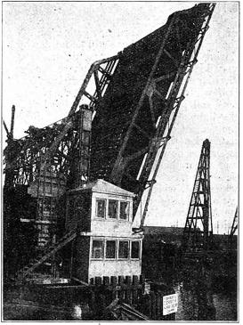
Electrically Operated Lift Bridge During Construction—View of Tower Which Contains Control and Motive Equipment.
