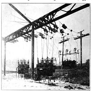
Control and Protective Apparatus for the 22,000-Volt Outgoing Lines.
