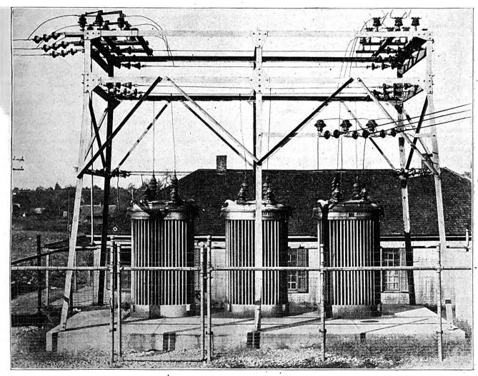
Fig. 2.—Modern Type of Outdoor Installation, Showing Three 150-Kv-a. Transformers With 2300-Volt Metering.
