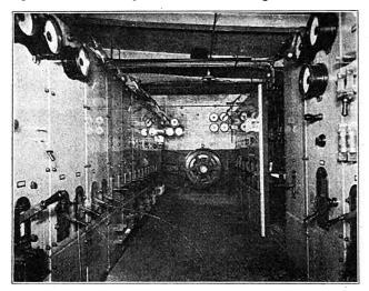
Fig. 2.—View in Central Substation, Showing Motor Control Panels and Distributing Boards—A 150-Hp. Motor Is Also Shown.
