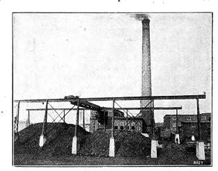
Fig. 2.—View of Installation Showing Transfer Crane Equipped with Grab Bucket Hoist. This Plan Provides for Future Extension.
