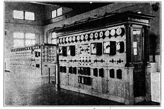
Five-Panel Switchboard Controlling High-Tension Lines and Transformers—14-Panel Board in Background.
