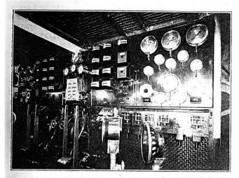
Main Switchboard and Control Apparatus Through Which Current Passes to the Propeller Motors.
