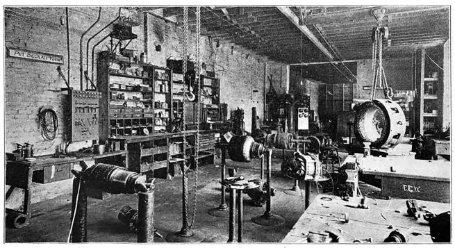
View of Squire Electric Co. Shop, Kansas City, Mo., Showing Longitudinal Overhead Holst Track, in the Path of Which Are Set the Winding Racks. At the Left is a Testing Rack of 5000-Voit Capacity.
