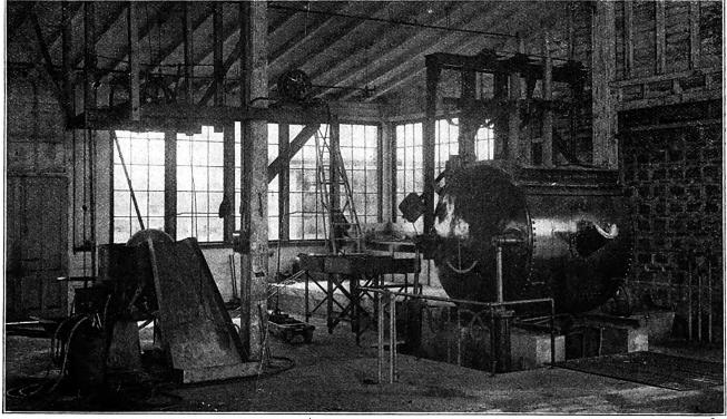
A 2-ton Greene Electric Furnace for Making Steel Castings in Foundry of Lamb Machine Co., at Hoquiam, Wash.
