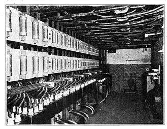
Fig. 3.—Rear View of Motor Control Panels in the Central Substation, from Which Nearly All the Motors Are Controlled.
