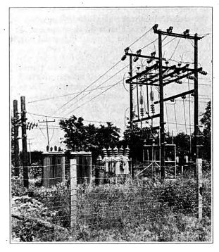
Economical and Simple Construction for 33,000-Volt Outdoor Substation and Switching Center.
