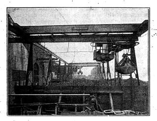
Fig. 3.—Shepard Transfer Cranes Equipped with Grab Bucket Hoists Over Coal Storage Pile. Coal Shown in Background in Barges and Transferred to Storage.
