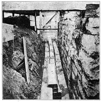
Fig. 4.—Four-part Duct as Used in Horizontal Duct Line After Single Duct Emerges From Riser From Tunnel.
