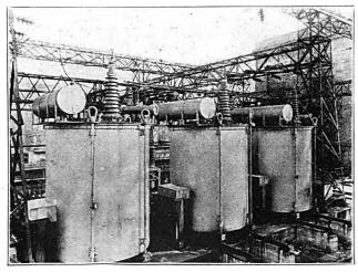
Fig. 4.—Transformers With Oil Conservators at the Windsor Power Plant of the American Gas & Electric Co.
