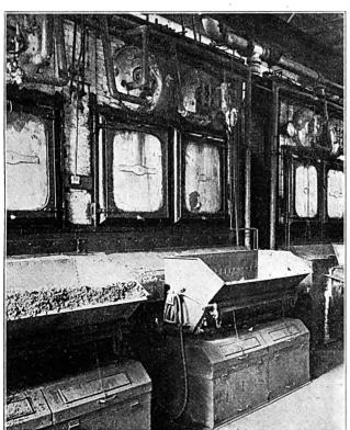
Windows in Stoker Casing as Used Successfully with Chain-Grate Stokers Using Forced Draft and High Rates of Combustion.
