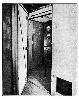
Fig. 2.—Asbestos Housing for 100-Kv-a. Static Condenser installed Indoors.
