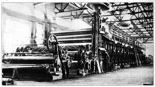
Front of 174-in. Paper Machine, Driven by 600-hp. Motor.
