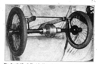
The Small "Dey" Electric Motor Is Mounted on the Rear Axie.
