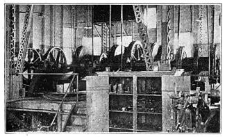
Five-Drum Winch Used for Operating Spuds, Cutter Head and Headlines.
