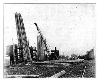
Plant of Western Cedar Pole Preservers, Sand Point, Idaho, Showing Locomotive Crane in Service and Two Loads of Poles Receiving "B" Treatment.
