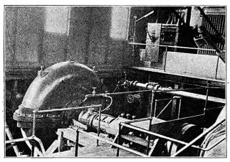
Interior of Oakland Dredge, Showing Pumps and Power Transformers.
