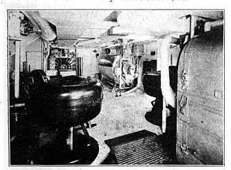
View in Laundry, Showing Motor-Driven Washing Machines, Electric Dryer and Electric Sterilizer.
