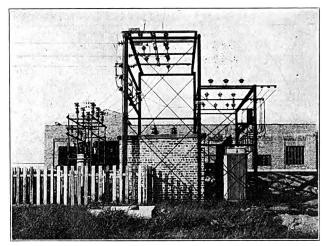
Fig. 4.-1200-kw. 33,000/2300-Volt Three-Phase Substation.
