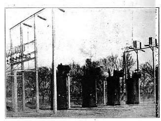
Fig. 5.—Outdoor Installation of Conservator-type Transformers of the Virginia Rallway & Power Co., Richmond, Va.
