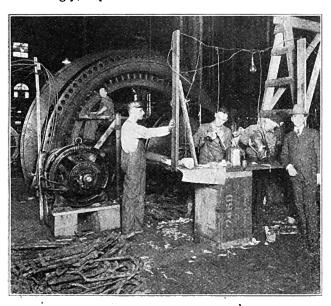
· Improvised Work Bench Used by Contractor in Reinsulating Stator Colls of Alternator.
