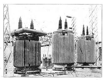
Fig. 3.—Initial Installation of Transformer Provided With Oil Conservator at Laurinburg, N. C.
