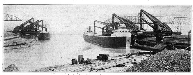
Eight Electrically Operated Ore Unloaders at Ashtabula, Ohio—These Docks Have an Unloading Capacity of 76,000 Tons of Ore
