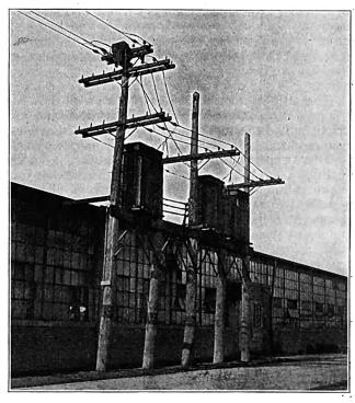
Three 200-kv-a. Transformers Mounted Upon Platform with Automatic Oil Switch and Control Ropes.
