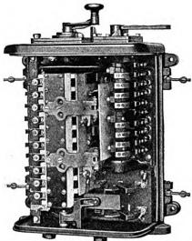
New Two-Motor Storage Battery Locomotive Controller—Cover Removed to Show the Two-Cylinders.
