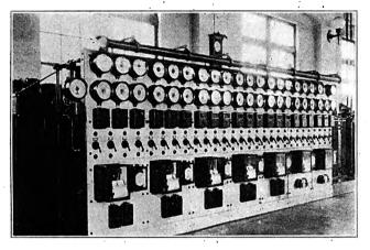
Seven-Panel Feeder Switchboard Installed in Nisqually Substation, Tacoma, Wash.
