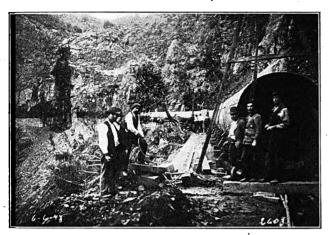
Pangai Hydroelectric Development-One of the Riveted Steel Sections of the Pipe Line Which Were installed on All Curves of Less Than 375-Ft. Radius.
