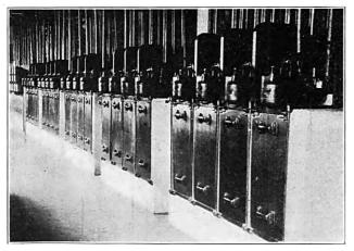
Five 4000-Volt, 600-Ampere, Four-Pole Oil Switches on Light and Power Lines.
