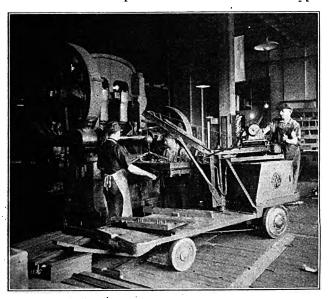
An Electric Truck With a Crane Attachment Can Be Used for Lifting Heavy Materials Onto Machines.
