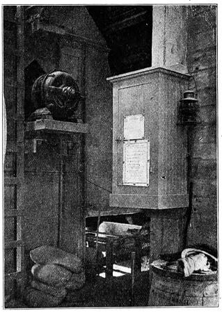
Fig. 5.—7½-hp., 680-r.p.m., 440-volt, 60-cycle Motor Driving Clinker Elevator.
