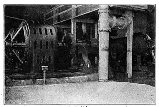
Motor-Generator Set, the Driving Unit of Which is a 725-hp. Synchronous Motor.
