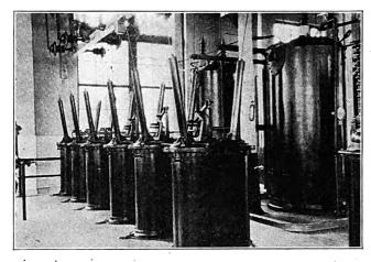
Three-Pole 60,000-Volt, 300-Ampere Oll Circuit-Breakers on Incoming Lines-Transformers in Background.
