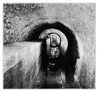
Fig. 2.—Duct Line Laid and Cemented in Tunnel of Concrete.
