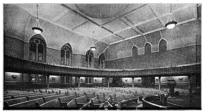
Fig. 4.—General View of the Auditorium, Showing Both Ceiling and Walf-Lighting Units.
