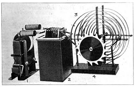
Figs. 1 to 4.—Thordarson Radio Transformer, Condenser, Oscillation Transformer and Rotor for Spark Gap. .
