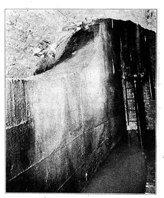
Fig. 5.—Duct Line Where Horizontal Run Changes to Vertical.
