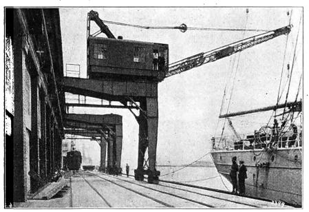
Fig. 1.—The First of Four Semi-Portal Cranes In Operation with Boom in Lowest Position.
