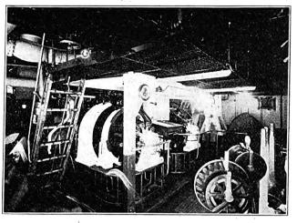
Two Main Exciter Sets for Turbogenerators that Supply Current to the Propeller Motors.
