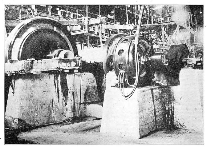
View of Tube-Mill Unit in Mill of Tonopah-Belmont Development Co., Showing 100-Hp. Motor Drive, With Morse Chain Transmission.
