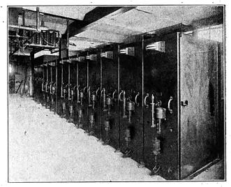
Fig. 2.—Truck Type Panels for 2300-Voit Single-Phase Feeders.
