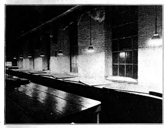
Fig. 6.—Inspectors' Tables Effectively Lighted to High Intensity so That Any Defect in the Cloth Can Be Detected
