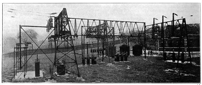
Another (Nearer) General View of North Substation, Showing Initial Installation of Three of the Big Transformers and Substation Building at Right.
