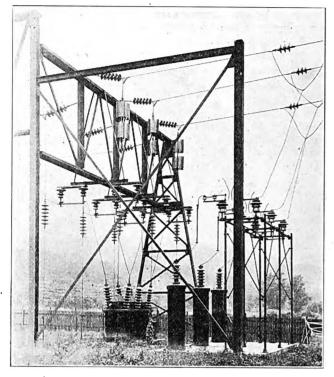
The 66,000-Voit incoming Line With Kickoffs, Lightning Arresters, Choke Colls, Circuit-Breakers and Disconnects.
