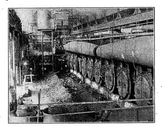
Fig. 1.—Grab Bucket Hoist Shown Inside Power House and Placed Where Coal is Discharged for Firing Bollers.
