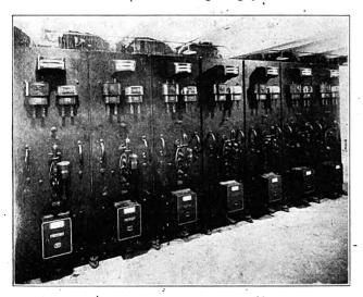
Fig. 3.—Truck Type Panels for 6600-Volt Three-Phase Feeders.
