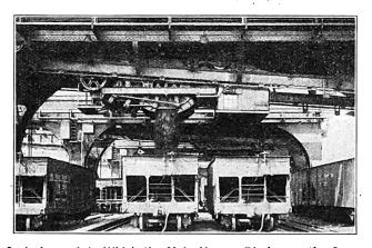
Scale Larry Into Which the Main Hopper Discharges the Ore— This Larry Weighs the Ore and Discharges It Into Cars or Into Storage.
