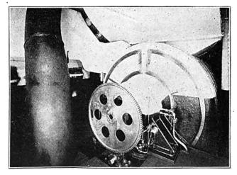
Cne of the Two Main Turbogenerators for Producing the Polyphase Current for the Propeller Motors.
