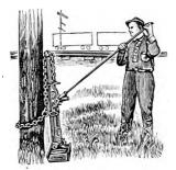
By pulling and straightening poles in a fraction of the time and with one-third of the men required to do the work in the usual way, this exclusive Simplex tool has established a record for economy and efficiency heretofore unattainable in this work. Adopted as standard equipment by hundreds of Telephone Companies.
