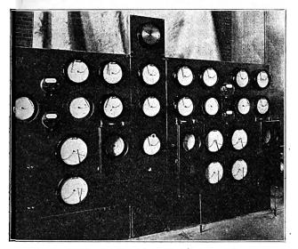
Board Containing Full Equipment of Instruments by Which Priming Could be Detected.
