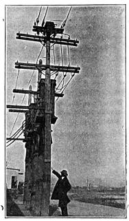
End View Showing Oil-Switch Control Ropes, Lightning Arresters and Conductor Arrangement.
