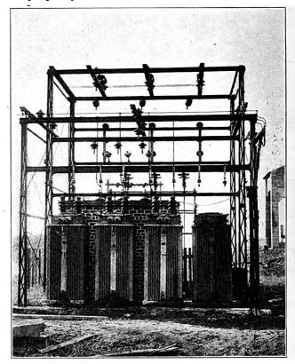
Fig. 2.—Substation Tapping Power Line Giving Service to a Coal Mine Containing 900-kw. 33,000/2300-Volt Three-Phase Transformer.
