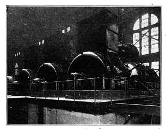
Fig. 3.—Close-Up View of 70,000-kw., Triple-Compound Turbine, Largest in the World.
