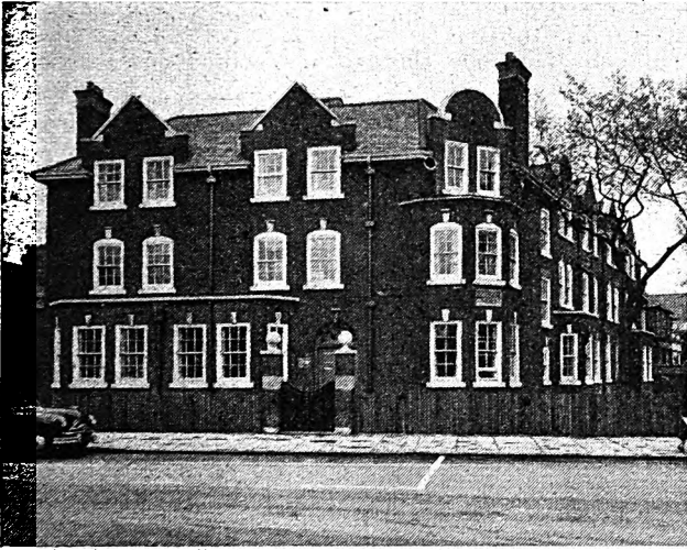
Fig. 1—Exterior of building.
