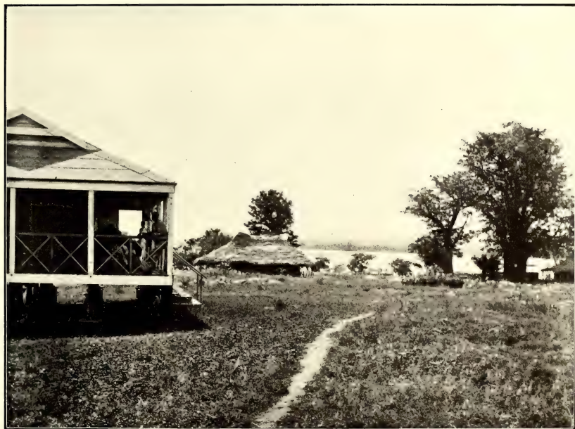
PORTION OF THE BARRACK SQUARE AT LOKOJA, SHOWING A EUROPEAN OFFICER'S BUNGALOW, AND TWO OR THREE NATIVE HUTS CLOSE BY. TO THE RIGHT IS A STACK OF ANT-PROOF PILES, SIMILAR TO THOSE ON WHICH THE BUNGALOWS ARE BUILT. THEY ARE PARTIALLY OVERGROWN WITH GRASS. THE TRAPS CONTAIN WATER WITH MANY Anopheles LARVAE
