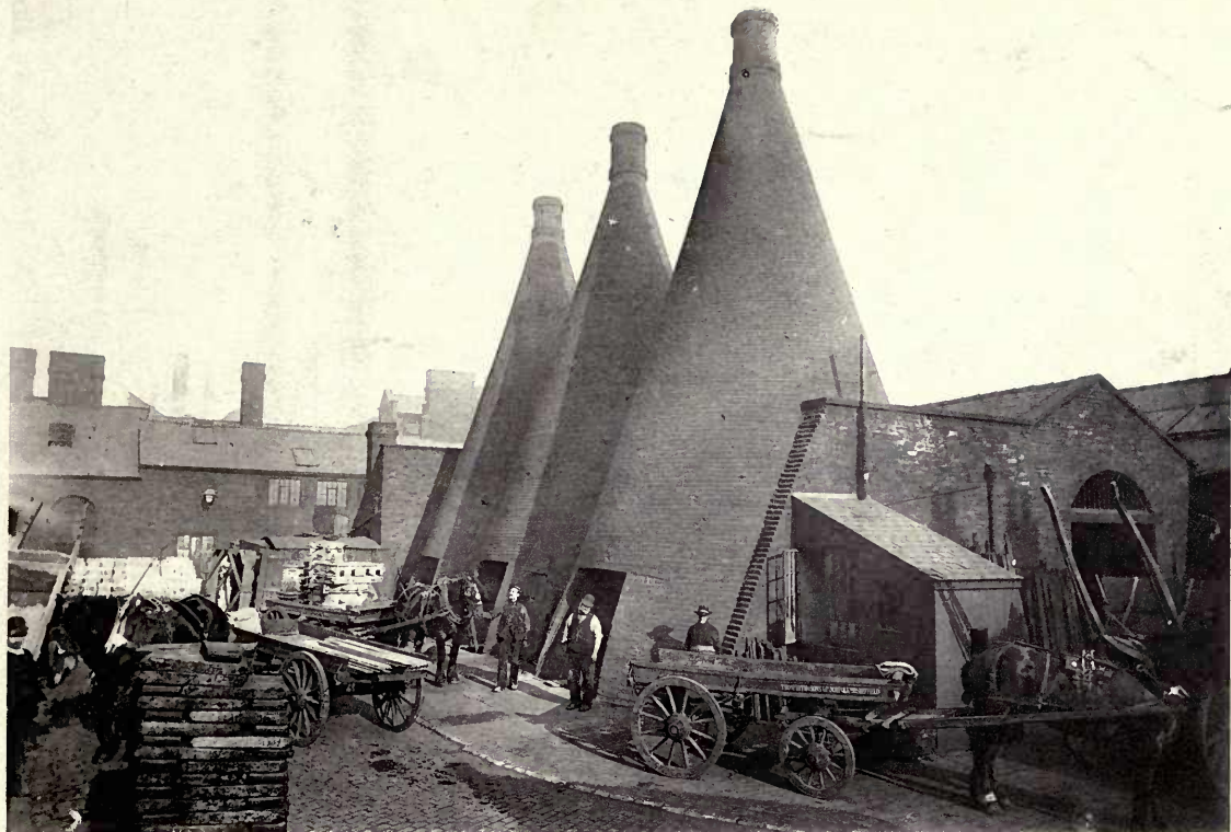
EXTERIOR VIEW OF CONVERTING FURNACES AT NORFOLK WORKS.
