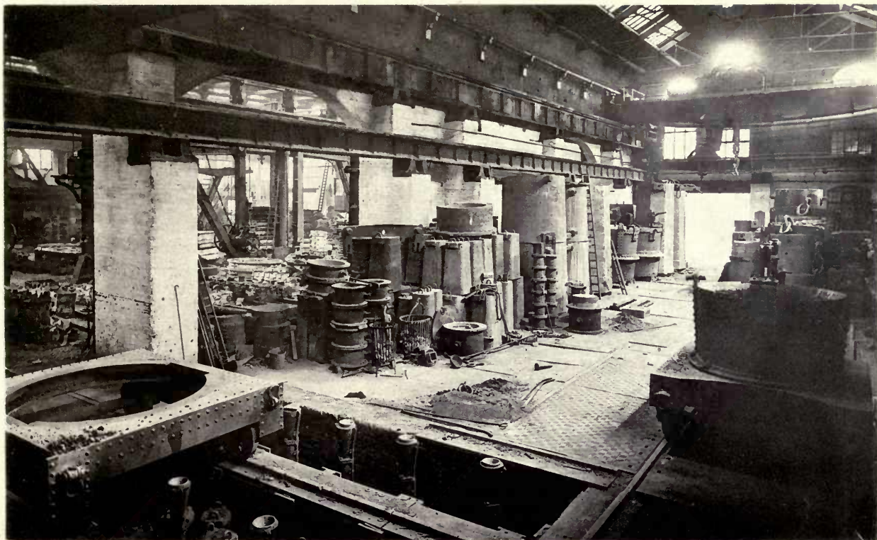
LARGE INGOT CASTING SHOP, WITH 100 TON TRAVELLING CRANE, AT NORFOLK WORKS.
