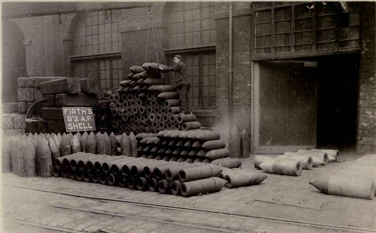
GROUP OF 9.2in. CAPPED A.P. SHELL PARTIALLY MACHINED.
