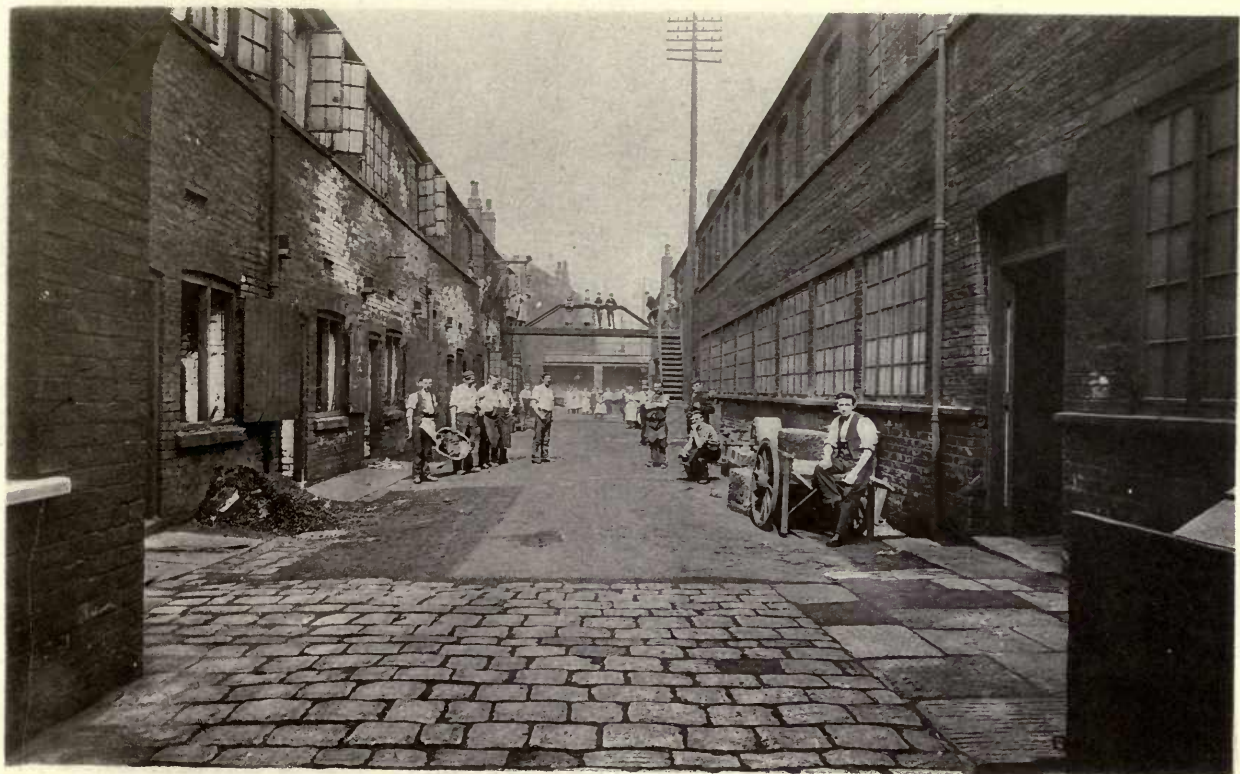
INTERIOR, OLD FILE FACTORY..
