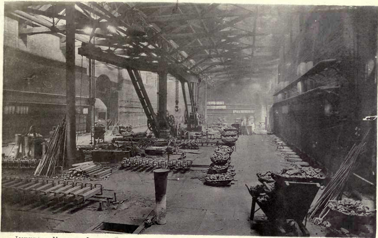
INTERIOR VIEW OF LARGE CRUCIBLE STEEL 100-HOLE MELTING FURNACE AT NORFOLK WORKS. 163 feet long x 70 feet wide. Area 1,269 square yards.
