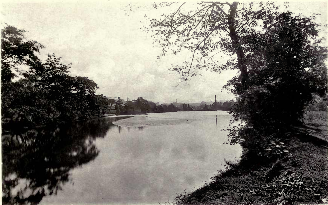
DAM AT CLAY WHEEL FORGES.
