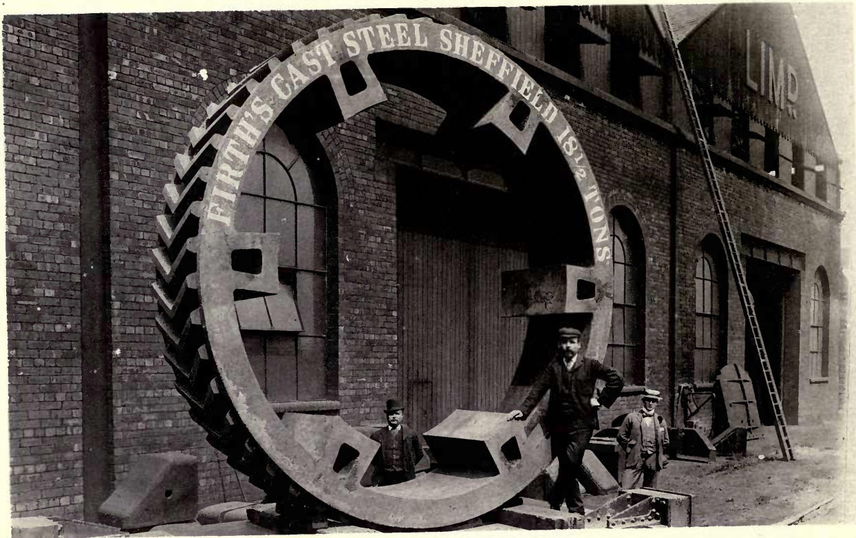
STEEL CASTING, WEIGHT 18½ TONS.
