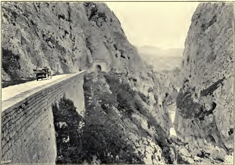
The Tunnel on the Furlo Pass
