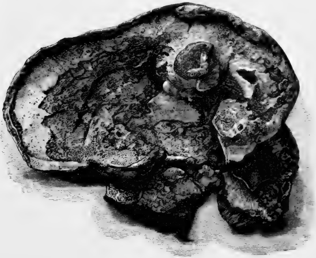
FIG. 21.—Portion of the mycelium of Merulius lacrymans removed from the surface of a beam of wood. This cake-like mass spreads over the surface of the timber, to which it is intimately attached by hyphæ running in the wood-substance. Subsequently it develops the spore-bearing areolæ near its edges. The shading indicates differences in colour, as well as irregularities of surface.
