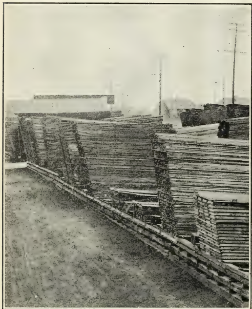
FIG. 37.—The latticed type of built-up plank foundations. This is an improvement over the solid type, as it allows better ventilation beneath the piles.
