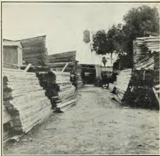
FIG. 33.—A very congested retail yard at New Orleans, La., showing lumber temporarily placed on the ground in solid piles. This is a bad practice, because under such conditions decay may start in a very short time.
