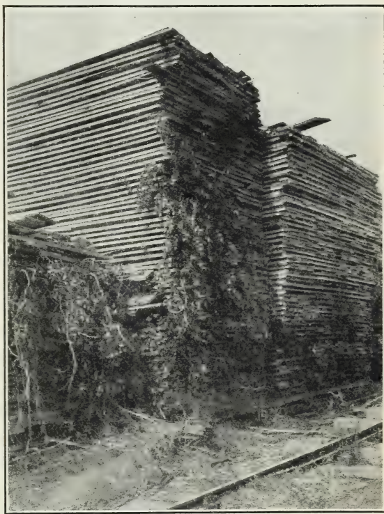
FIG. 13.—Vines growing over lumber piles. From a pathological standpoint this condition should be condemned, because the dense foliage prevents the lumber from rapidly drying out after rains, thus promoting decay.
