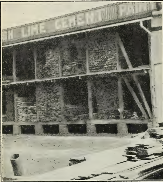
FIG. 31.—A retail shed in Tennessee, well roofed, provided with gutters, and set on brick piers with ample ventilation beneath from all sides.
