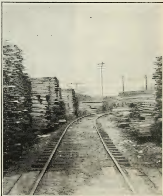
FIG. 15.—A clean, sanitary retail yard, having concrete foundations throughout and creosoted ties in the railroad track.
