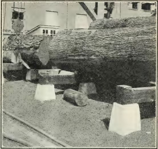
FIG. 18.—Pile foundations consisting of creosoted timbers resting on concrete piers in use at the Forest Products Laboratory, Madison, Wis. This is a very satisfactory type of foundation.
