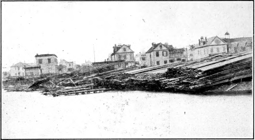
FIG. 2.—Lumber piled at the water's edge on the Atlantic coast. High waves sweep over this during storms, wetting the lumber and producing rot.
