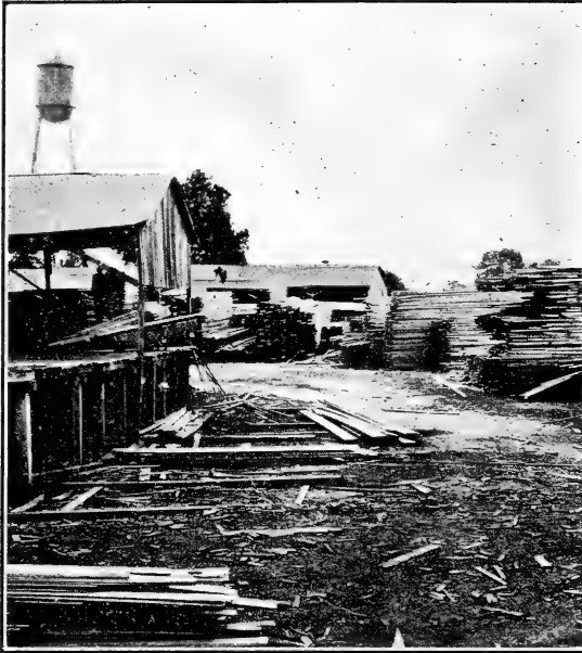
FIG. 7.—A small, very insanitary mill in Louisiana. The conditions at this mill are a disgrace to the lumber industry. Note the rotten, dilapidated tramway, the lumber stacks placed within 2 to 4 inches of the ground, and the debris scattered about and breeding infection.
