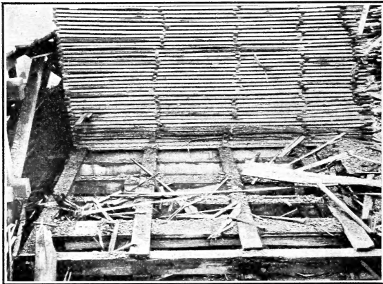
FIG. 3.—Silt deposited in the base of a lumber stack during a Mississippi River flood. This condition permits the lumber to rot rapidly.
