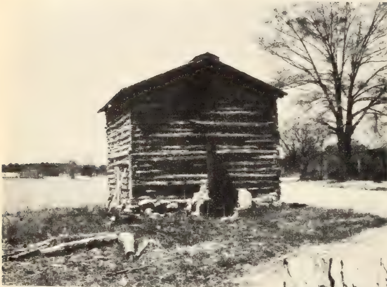
Figure 22.--The older type log curing barns had wood-burning fireboxes on the outside.
