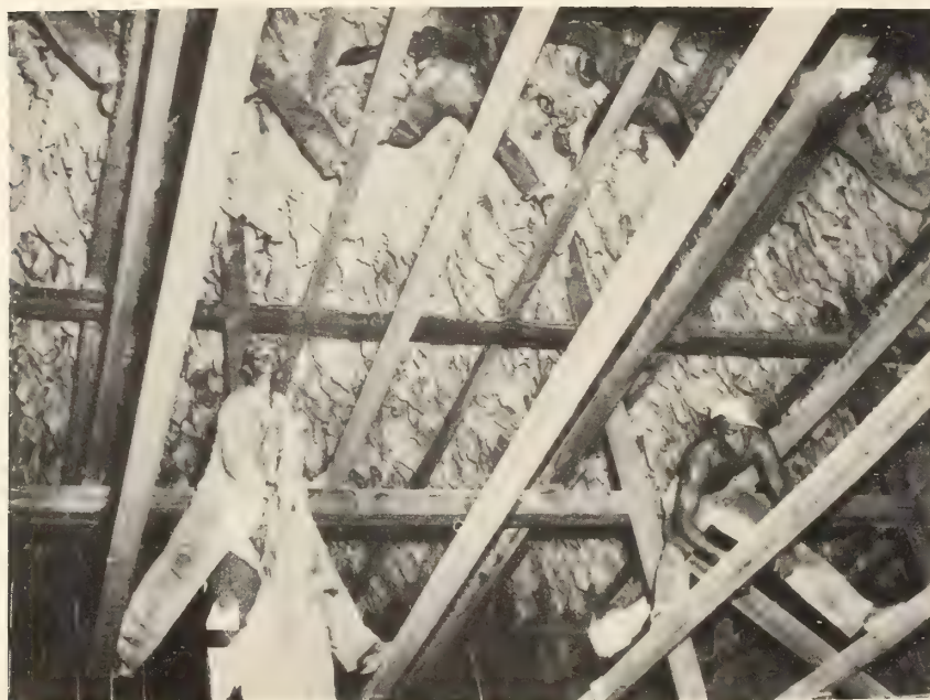
Figure 17.--Interior of burley curing barn showing green tobacco, which has been speared on sticks, being placed on the tier poles.
