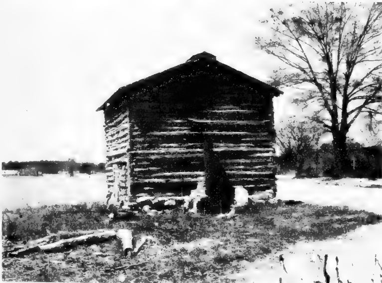
Figure 22.--The older type log curing barns had wood-burning fireboxes on the outside.
