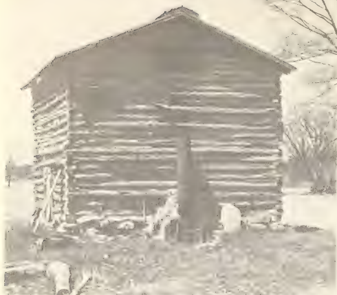
Figure 19.--The old flue-curing barns had wood burning fire boxes on the outside.
