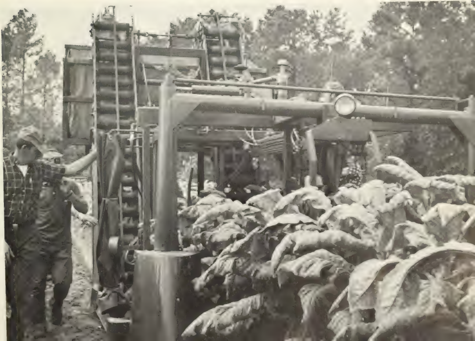
Figure 9.--Experimental version of mechanical harvester developed for flue-cured tobacco.
