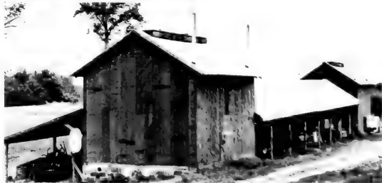
The majority of flue-cured growers still use this type of structure.
