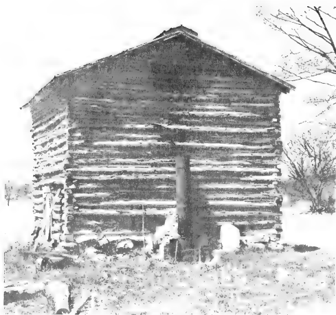
Figure 19.--The old flue-curing barns had wood burning fire boxes on the outside.
