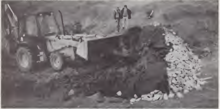
Construction of the sedge meadow dam. Photo by Elise Stevenson, November 1991.
